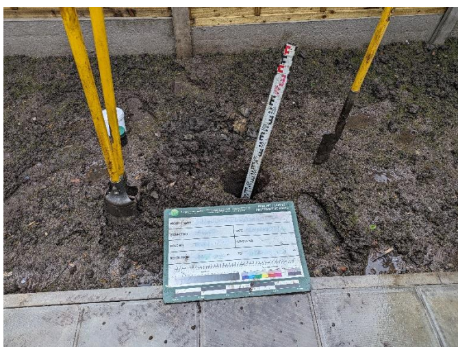
Hand dug pit HP1: Overview of excavation
