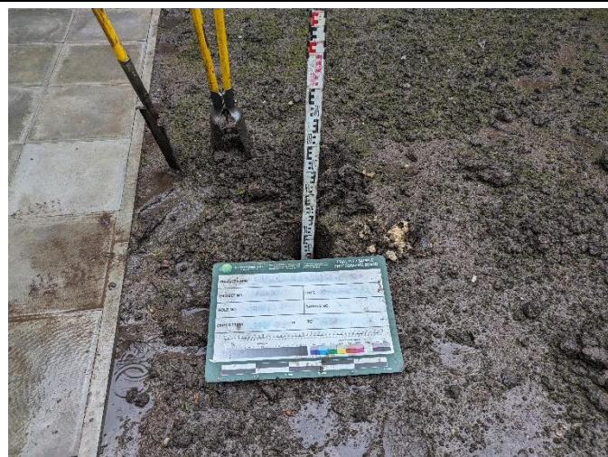
Hand dug pit HP2: Overview of excavation
