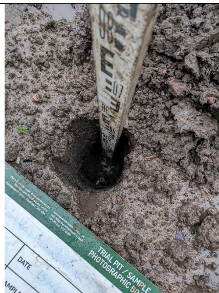
Hand dug pit HP8: Internal view of excavation
