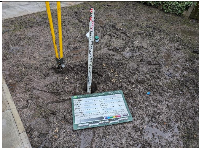
Hand dug pit HP4: Overview of excavation
