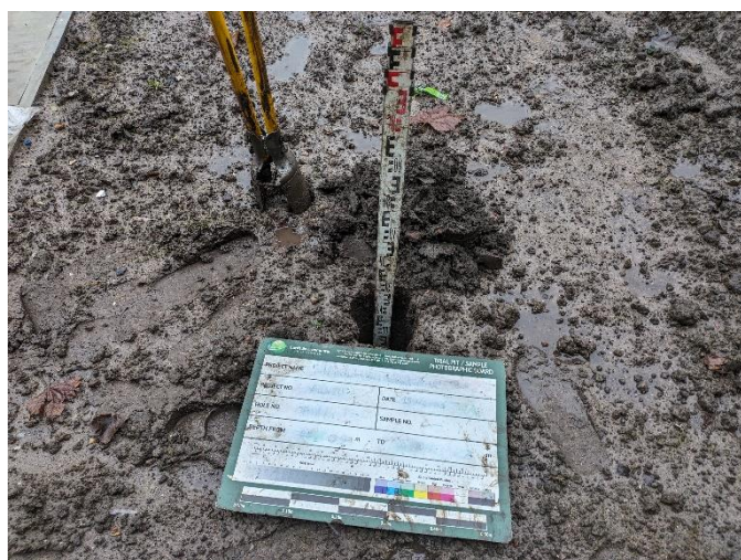
Hand dug pit HP8: Overview of excavation
