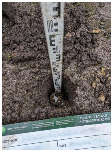
Hand dug pit HP2: Internal view of excavation
