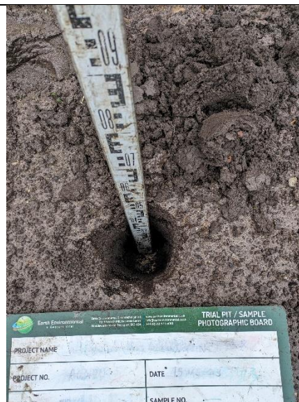
Hand dug pit HP6: Internal view of excavation
