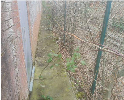
Photo 7: Railway boundary viewed north
