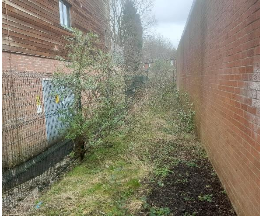
Photo 10: Northern boundary viewed east
