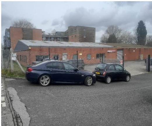
Photo 1: Site overview, front entrance
