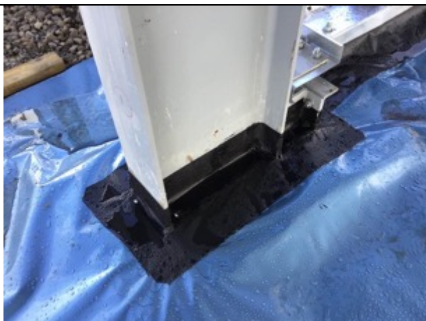
Block E sealed stanchion detailing
