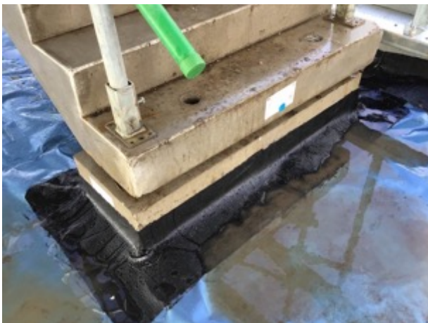
Block F sealed stair detail
