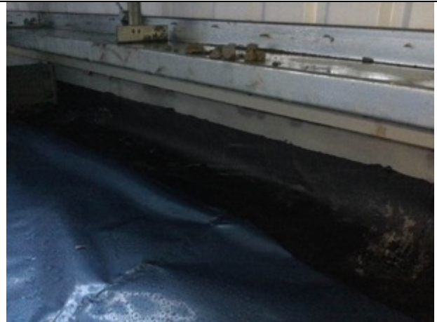
Retro detailing completed along the perimeter steel to Unit B office area.
