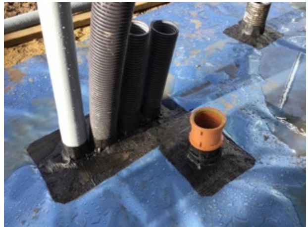
Block F sealed pipe penetrations
