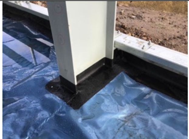
Block F sealed stanchion detailing
