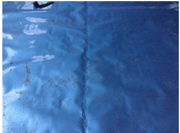
Overview to the hand welded lap joint to Unit A.
