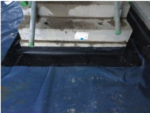
Stairwell detailing sealed with SAGM within Unit A.
