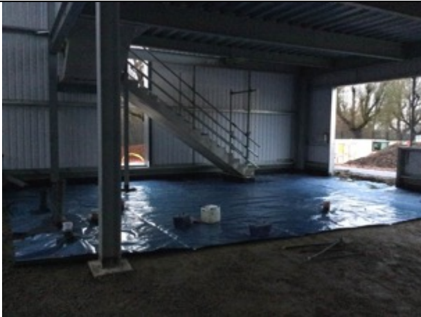
Unit A office area lined out.
