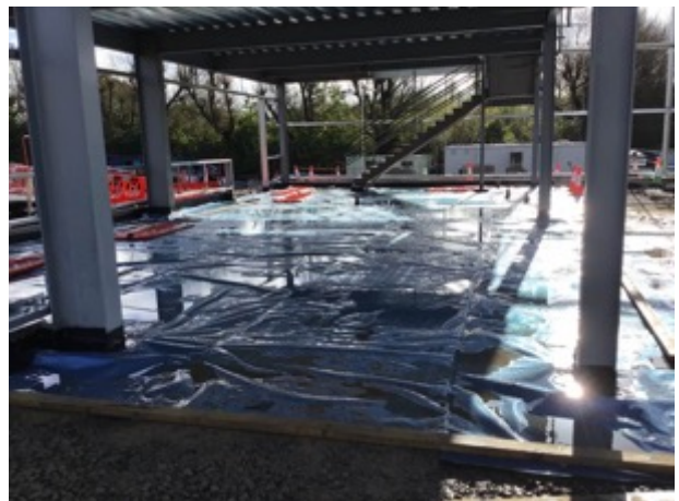
Block E office area overview
