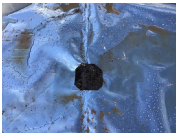
Sealed SAGM patch repair
