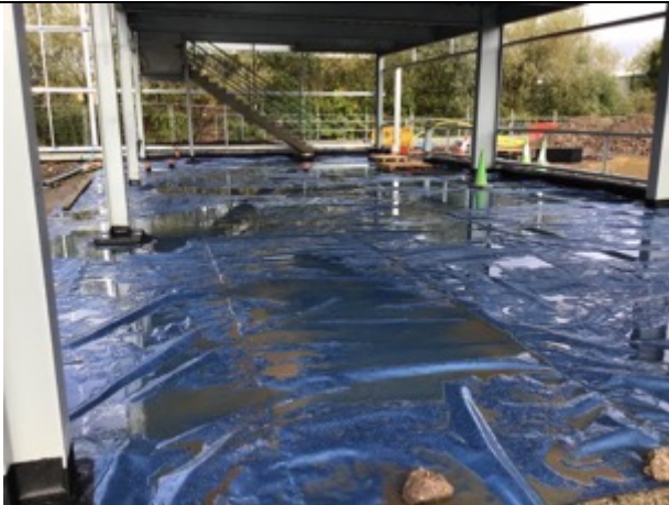
Block F office area overview
