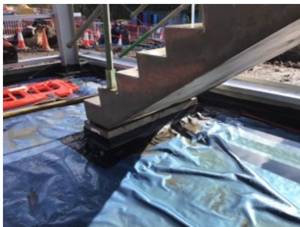
Block E sealed stair detail
