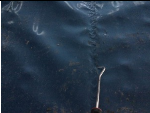
Pick testing along the lap joints to Unit B.
