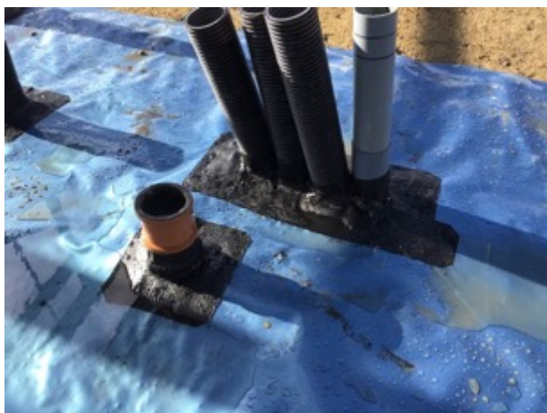
Block E sealed pipe penetrations
