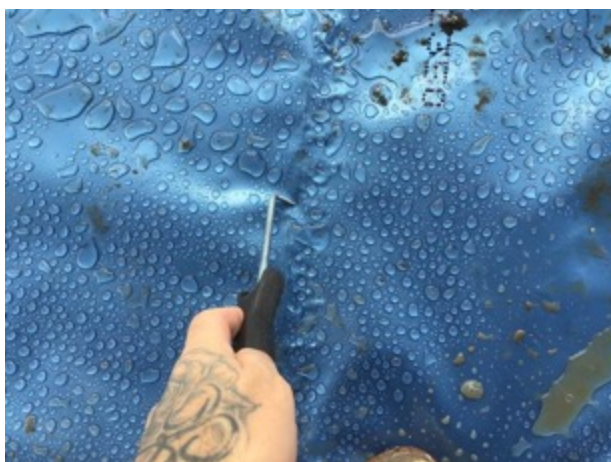
Pick test to sealed hand weld membrane joint
