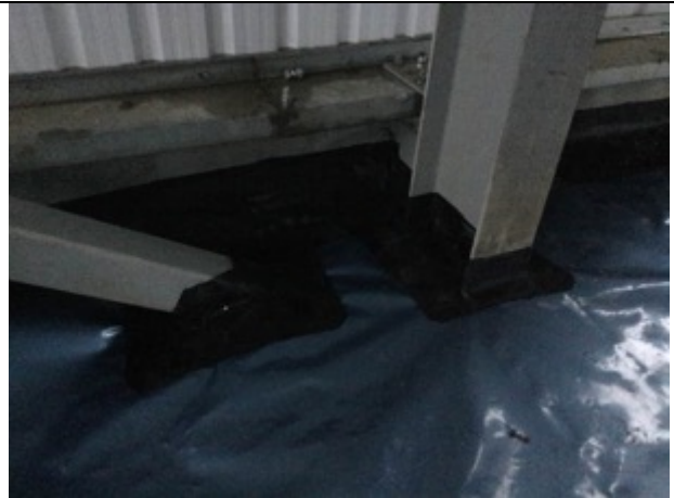
Steel stanchion detailing completed using SAGM.
