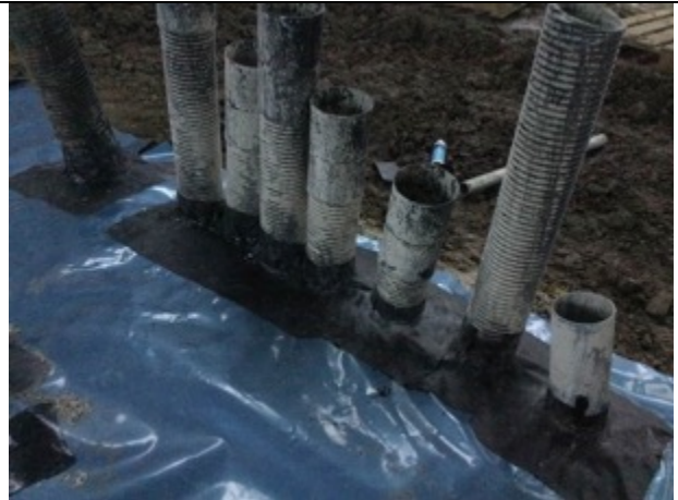
Multiple pipe penetration details sealed with SAGM to Unit D.
