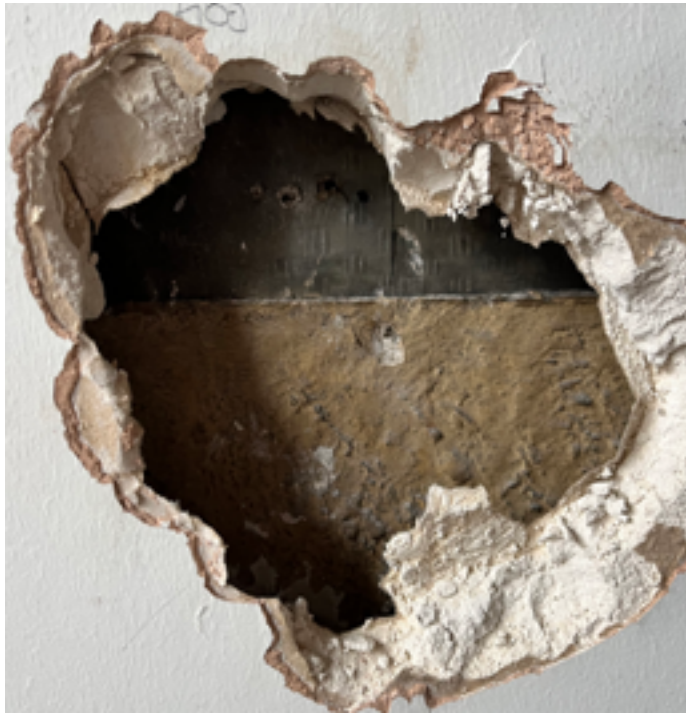
Figure 10 Photograph showing layers of wall finishes and overboarding within the unit
