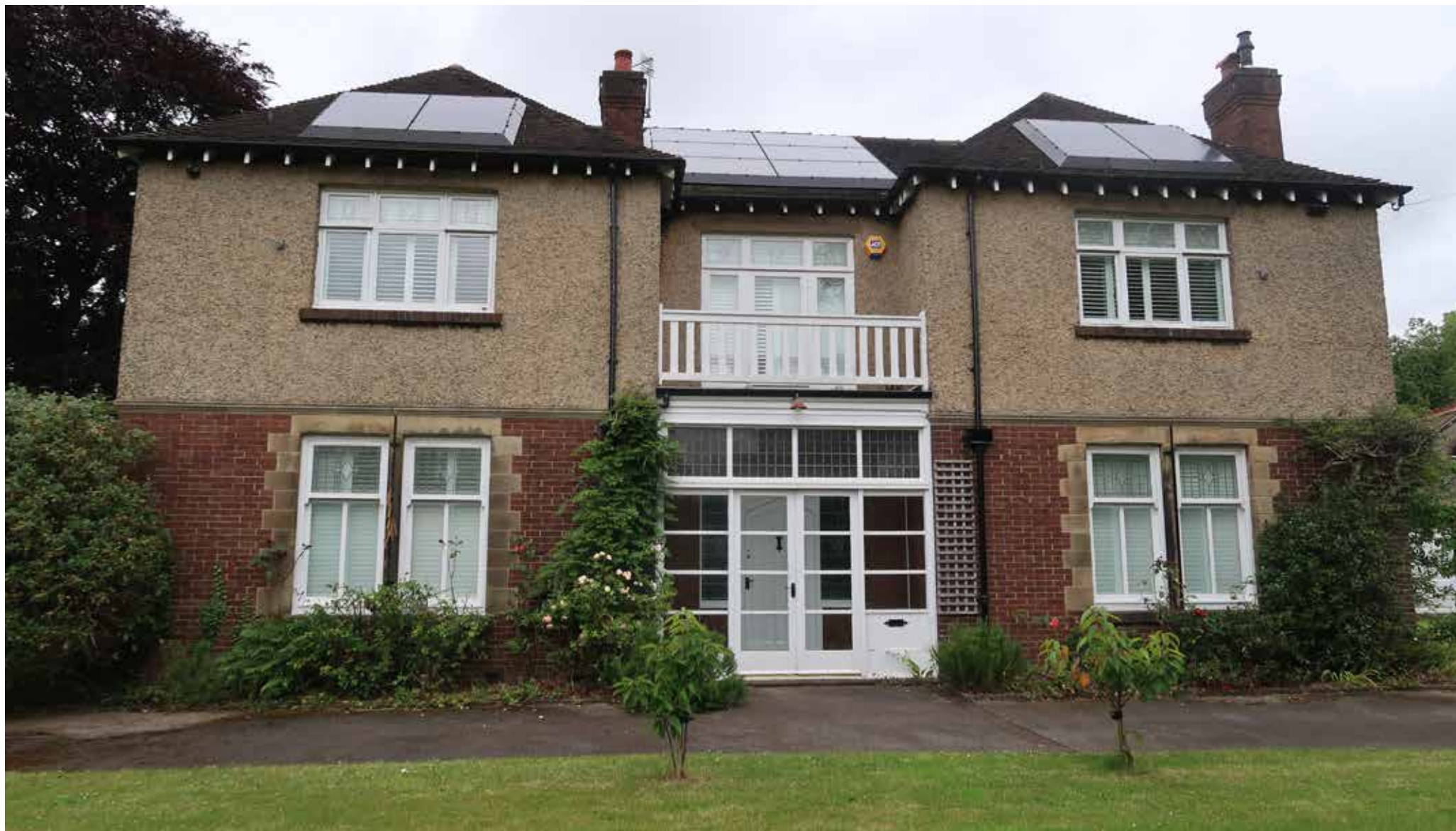
Exterior Principal Front.
