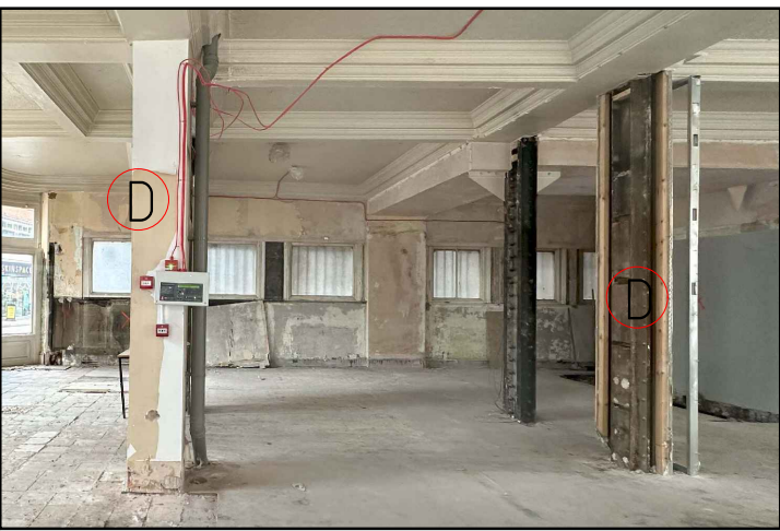
GROUND FLOOR COLUMN CASINGS
