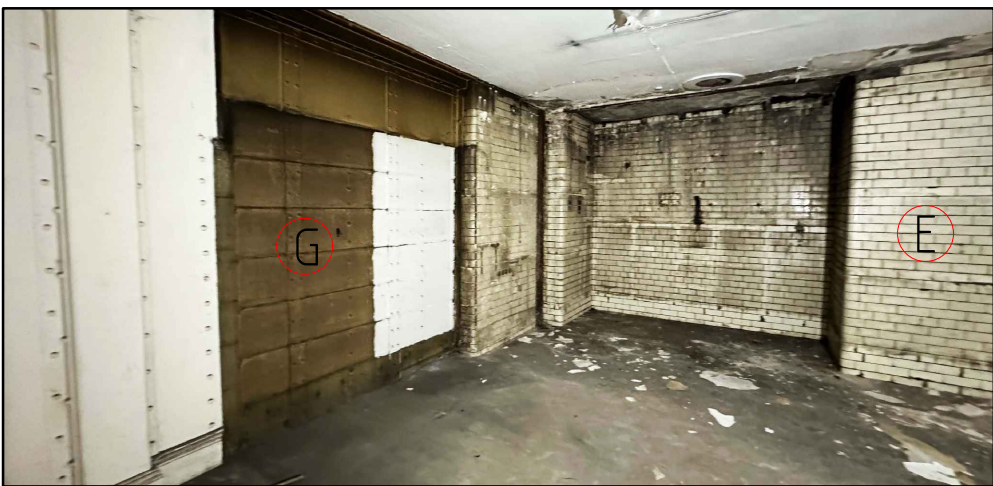
BASEMENT BRICK TILES AND METAL CLADDING
