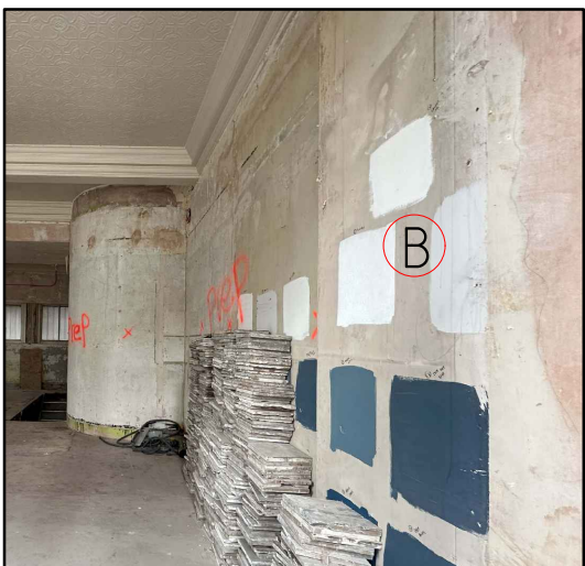
GROUND FLOOR PAINTED PLASTER WALLS
