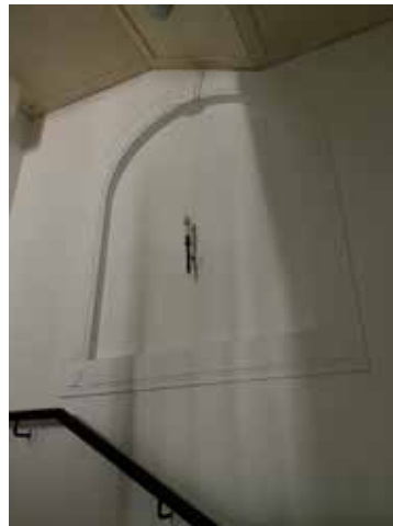
Plate 3.4.167 Niche on north outer wall at the quarter landings between ground and first floor
