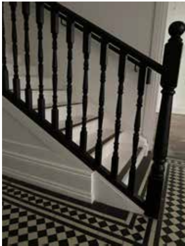
Plate 3.4.160 G.06 Staircase balustrading
