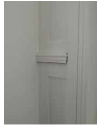
Plate 3.4.38 G.03 Wall moulding
