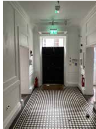
Plate 3.4.1 G.01 View to the front door to King Street
