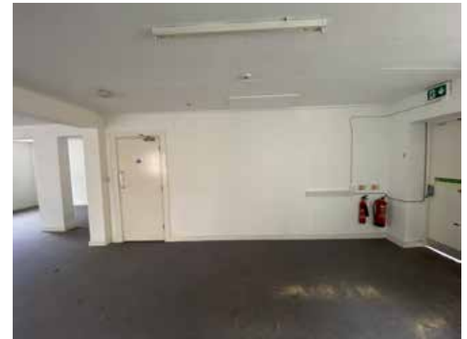
Plate 3.4.126 S.04 view to partition with stairwell
