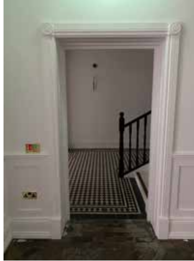
Plate 3.4.43 G.04 Architrave around opening to G.06
