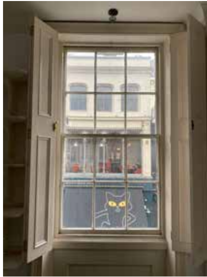
Plate 3.4.84 F.02 Sash window
