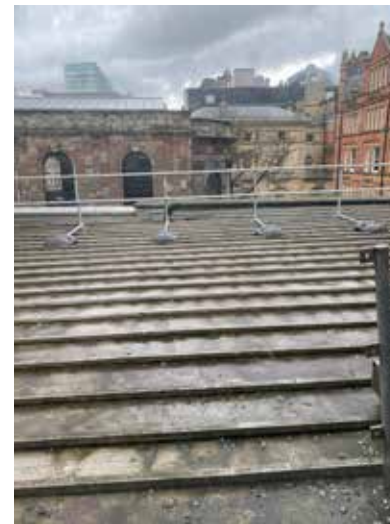
Plate 3.4.157 S.03 view north over the flat roof of the modern retail unit to St Ann's Church
