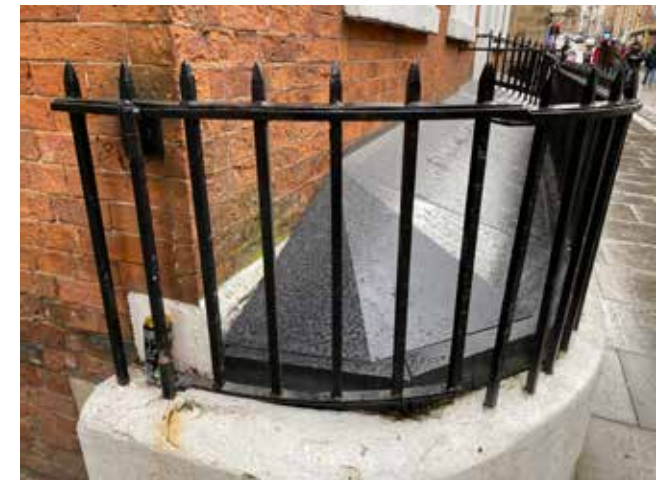
Plate 3.3.3 Rendered stone wall with railings
