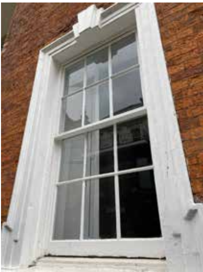
Plate 3.3.8 Example sash window detail (ground floor)
