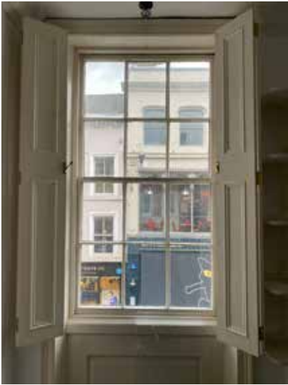
Plate 3.4.83 F.01 Sash window
