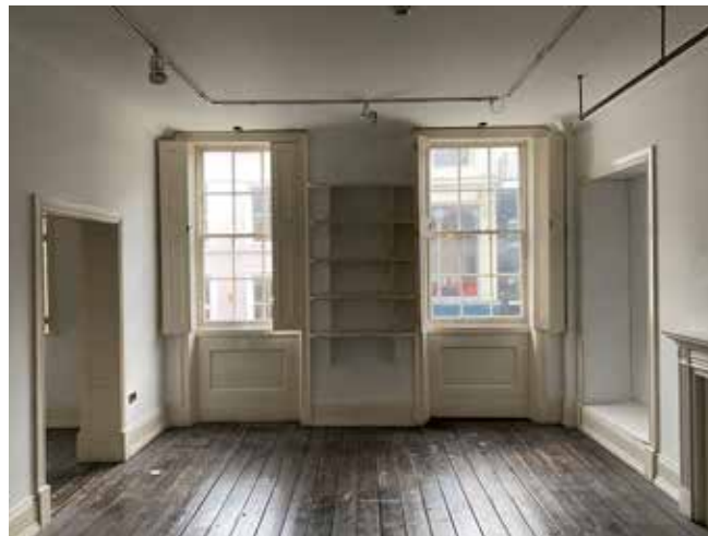
Plate 3.4.74 F.02 view to south outer wall
