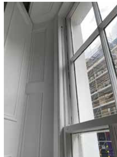
Plate 3.4.27 G.02 Sash window reveal detailing
