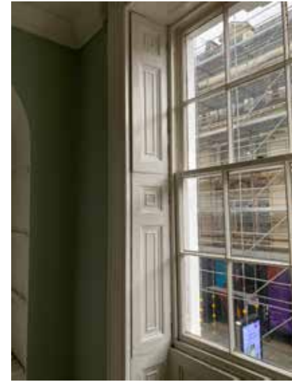
Plate 3.4.115 F.05 Sash window reveal with shutters in boxes
