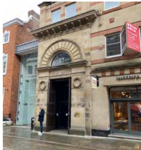
Plate 3.3.2 Remaining fragment of 19 th century bank extension at no.37 King Street
