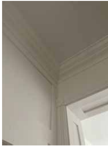
Plate 3.4.36 G.03 Cornice and detailing of architrave and panelling in aperture connecting G.02 and G.03
