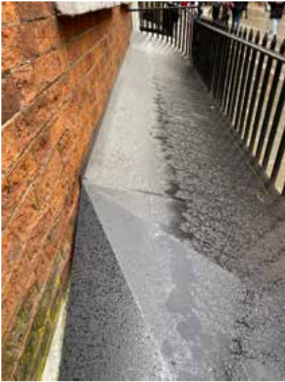
Plate 3.3.4 Lightwell with metal sheet cover
