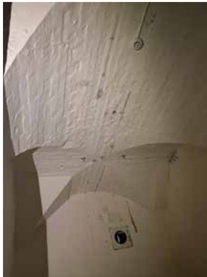
Plate 3.4.190 Brick vaulted ceiling in B.01
