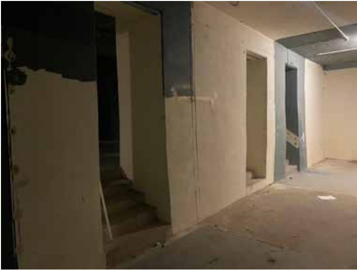
Plate 3.4.187 basement openings between the retail space and B.03
