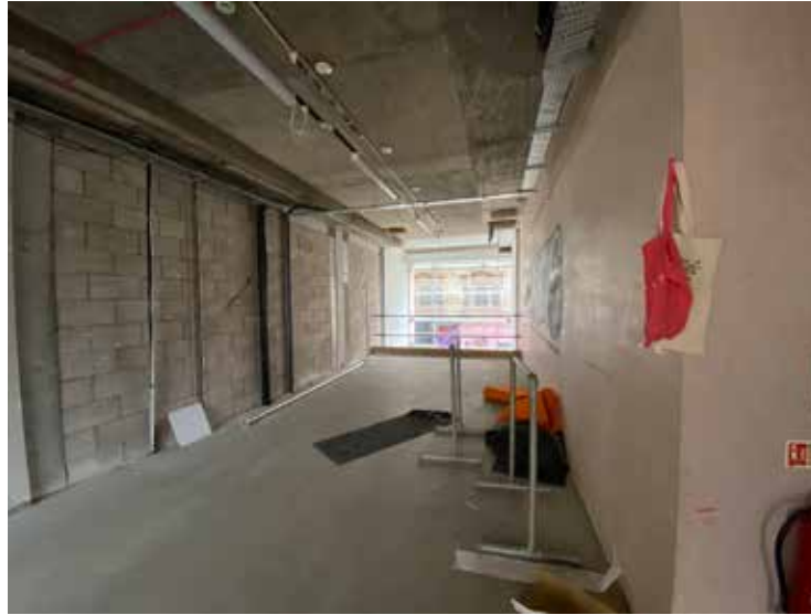
Plate 3.4.183 first floor east flanking wing
