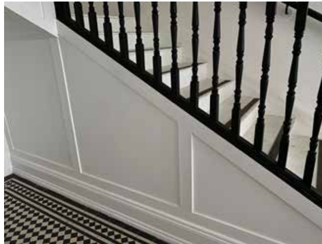
Plate 3.4.159 G.06 Staircase panelling and skirting
