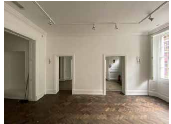
Plate 3.4.16 G.02 View to east partition wall (G.01 beyond)
