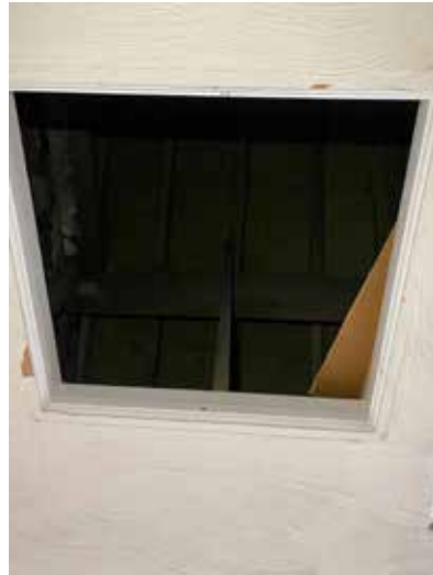
Plate 3.4.143 S.02 visible roof structure above ceiling
