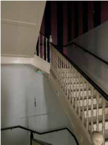
Plate 3.4.169 F.06 showing stair flights from first to second floor
