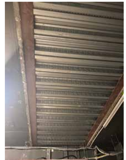
3.4.186 Ceiling in the rear part of the basement
