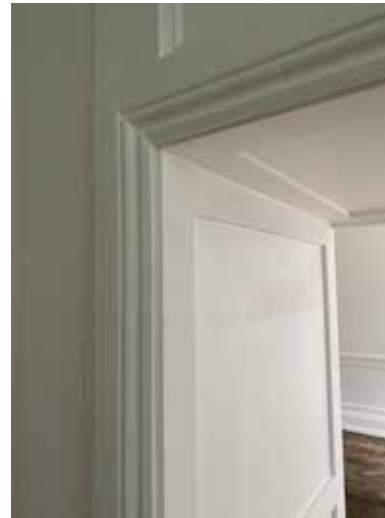
Plate 3.4.12 G.01 Deeper aperture reveal detailing (built out to joinery in G.05) between G.01 and G.05
