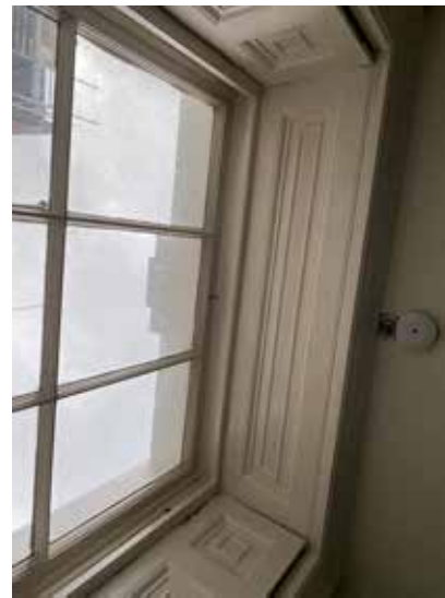
Plate 3.4.118 F.05 Sash window paneling
