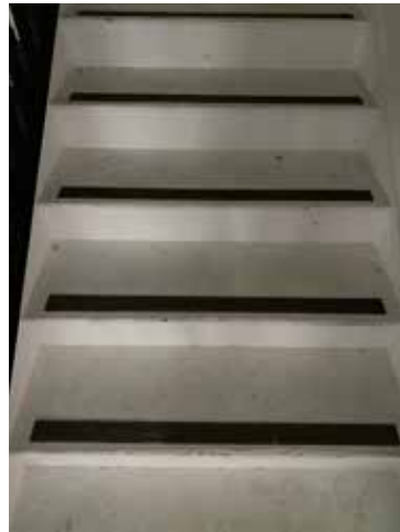
Plate 3.4.161 Lower flight of stairs from ground to first floor
