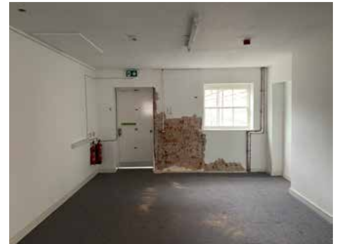
Plate 3.4.123 S.04 view to the north outer wall
