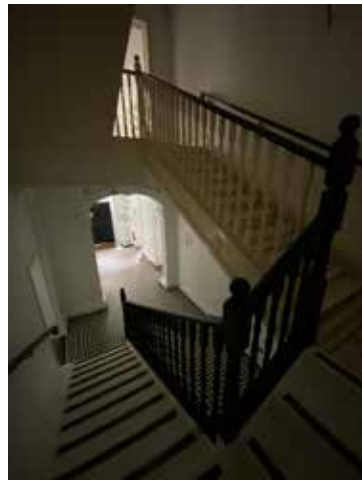
Plate 3.4.166 Staircase from ground to first
