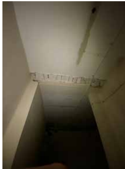
Plate 3.4.191 B.03 ceiling with visible brick
