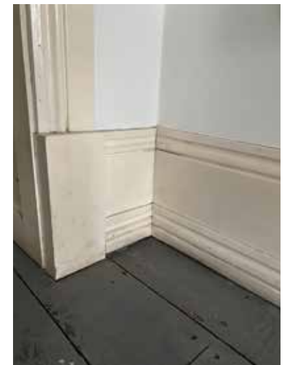
Plate 3.4.67 F.01 Skirting and architrave detailing
