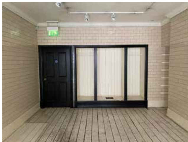
Plate 3.4.95 F.04 View to north outer wall
