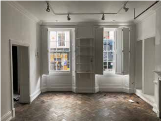
Plate 3.4.14 G.02 View to the south outer wall (King Street)
