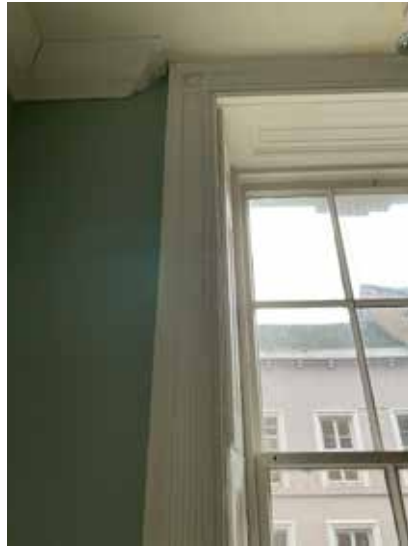
Plate 3.4.113 F.05 Sash window architrave
