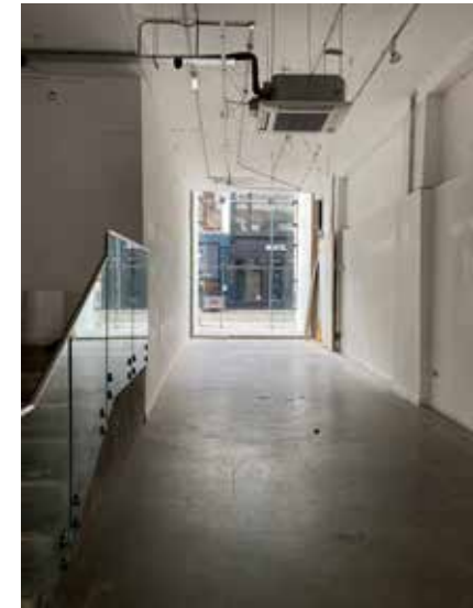
Plate 3.4.179 Ground floor west flanking wing
