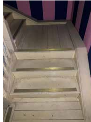
Plate 3.4.171 quarter landing from first to second floor
