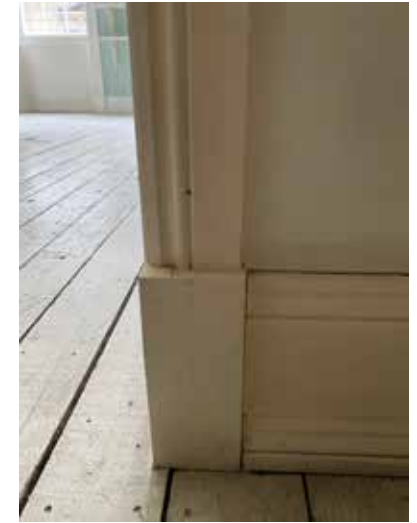
Plate 3.4.100 F.04 Skirting and architrave detail
