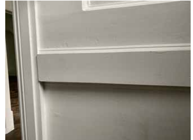
Plate 3.4.9 G.01 Dado and wainscoting detailing
