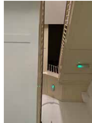
Plate 3.4.163 Underside of staircase
