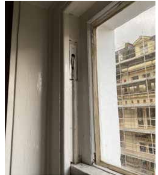
Plate 3.4.135 F.05 Sash window (front elevation) detail
