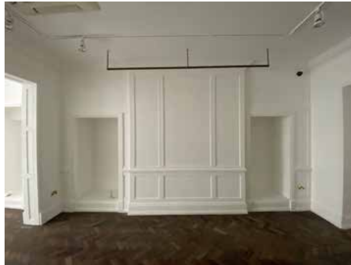
Plate 3.4.32 G.03 view to west outer wall
