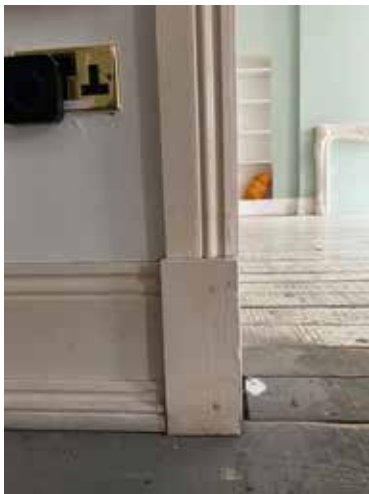
Plate 3.4.68 F.01 Skirting and architrave detail
