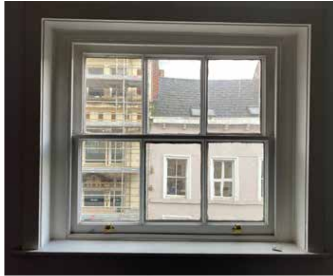
Plate 3.4.134 S.05 sash window in the front elevation
