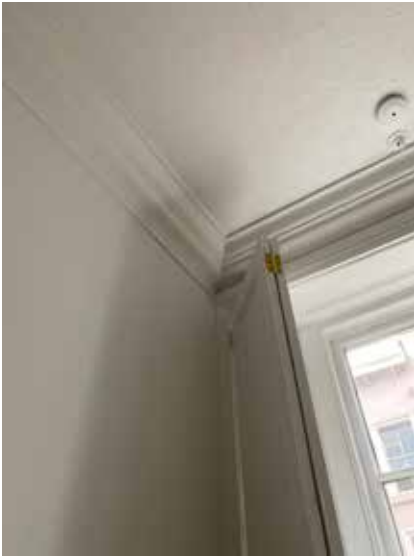
Plate 3.4.28 G.02 Window moulding and cornice detailing
