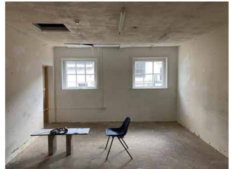
Plate 3.4.138 S.02 view to south outer wall
