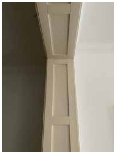
Plate 3.4.69 Paneling detail between F.01 and stairwell
