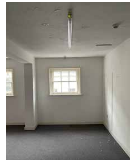
Plate 3.4.119 S.01 View to south outer wall
