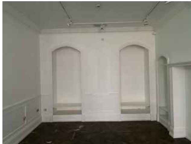
Plate 3.4.40 G.04 view to north wall
