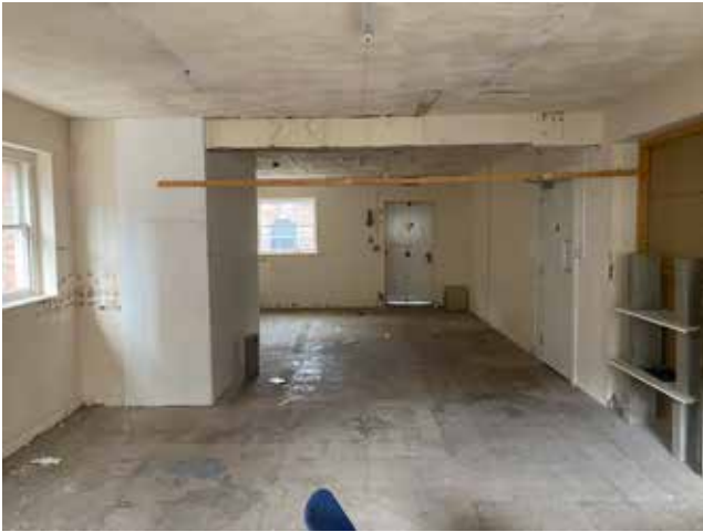
Plate 3.4.139 S.02 looking north to S.03
