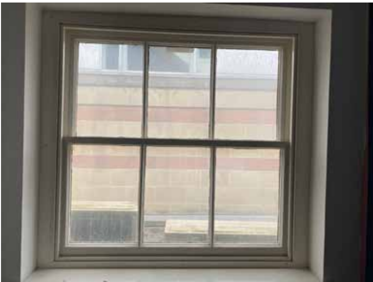
Plate 3.4.136 S.05 Sash window in the east return elevation
