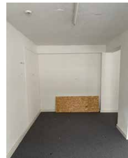
Plate 3.4.120 S.01 view to the blocked entrance to the stairwell
