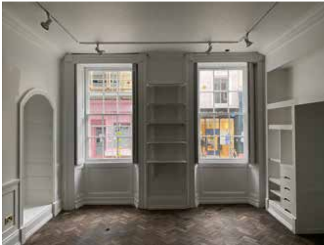
Plate 3.4.49 G.05 View to south outer wall
