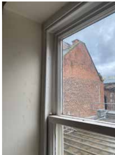
Plate 3.4.156 S.03 Sash window in the rear elevation detailing
