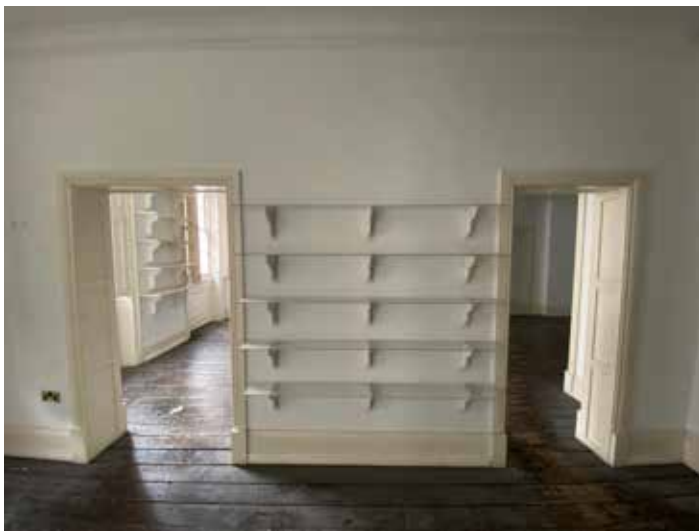
Plate 3.4.64 F.01 View to west partition wall
