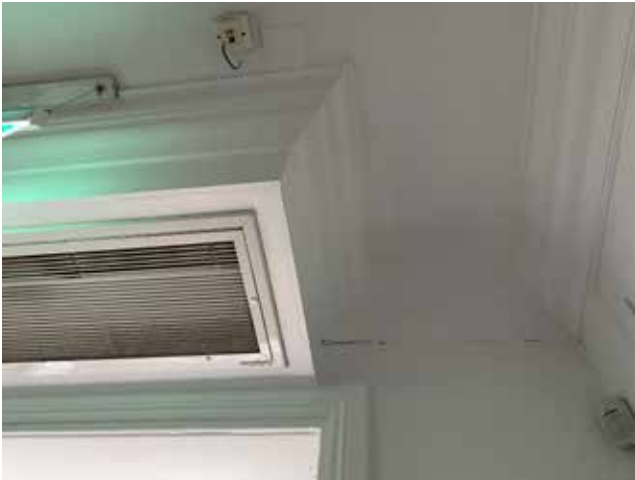
Plate 3.4.7 G.01 Cornice detailing around modern ventilation grille
