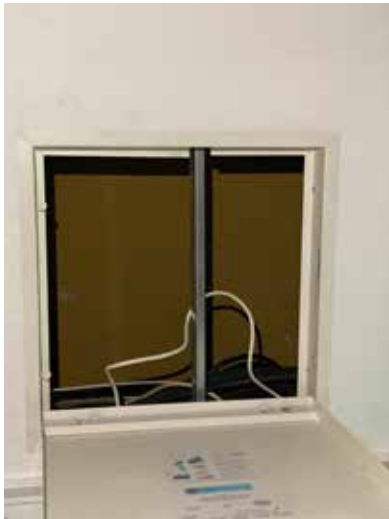
Plate 3.4.46 G.04 Open ventilation grille showing the ceiling suspended on metal hangars
