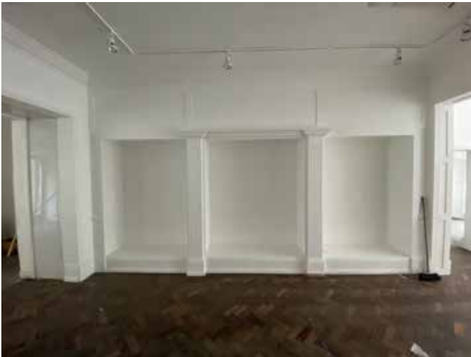
Plate 3.4.31 G.03 View to east partition wall
