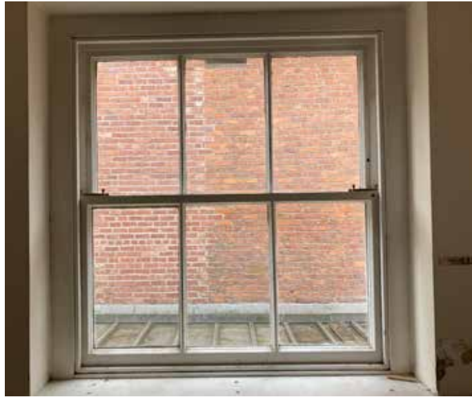
Plate 3.4.147 S.02 Sash window in the west return elevation
