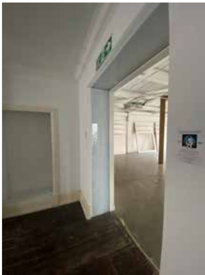
Plate 3.4.90 F.03 Aperture detail into modern retail unit
