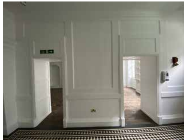
Plate 3.4.4 G.01 View to the east partition wall (G.05 beyond)
