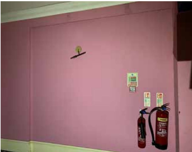
Plate 3.4.174 Blocked opening between the second floor landing and S.01
