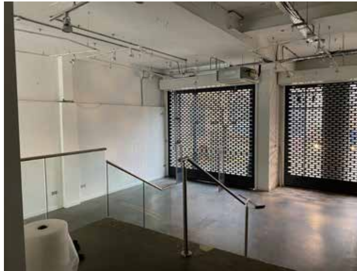
Plate 3.4.178 Ground floor retail unit to the rear (west side)
