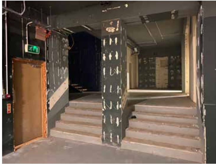
Plate 3.4.188 Large openings in the rear wall between the later retail space and B.02
