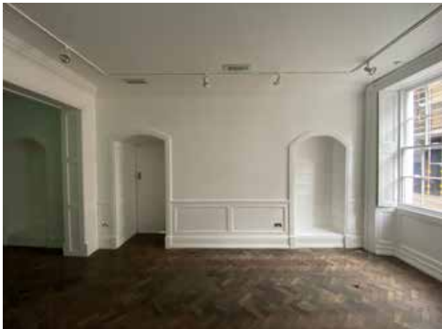
Plate 3.4.52 G.05 View to west outer wall
