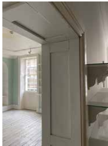
Plate 3.4.70 F.01 Paneling detail between F.01 and F.05
