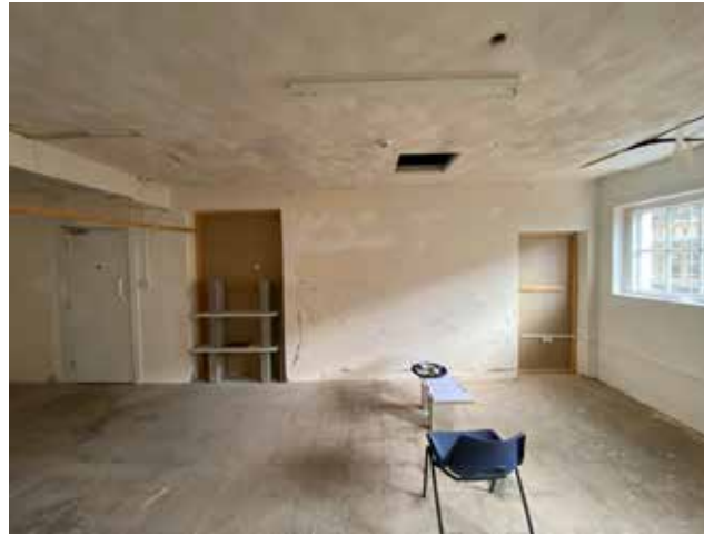
Plate 3.4.140 S.02 view to east partition wall (with S.01)
