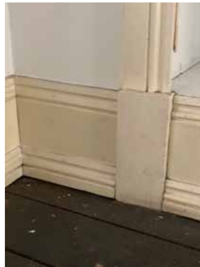
Plate 3.4.92 F.03 Skirting and architrave detailing
