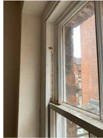
Plate 3.4.148 S.02 Detail of sash window in the west return elevation
