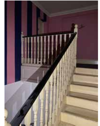
Plate 3.4.173 second floor landing
