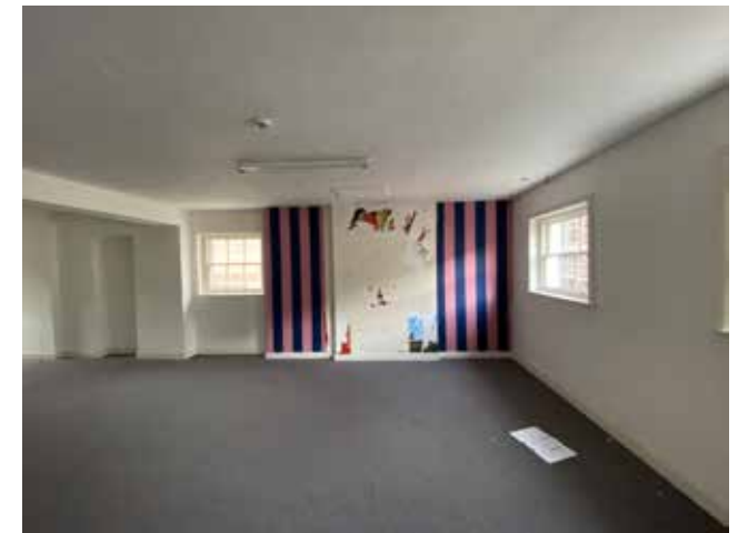
Plate 3.4.132 S.05 view to east outer wall
