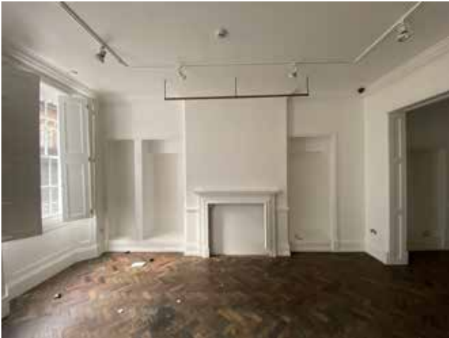
Plate 3.4.17 G.02 View to west outer wall
