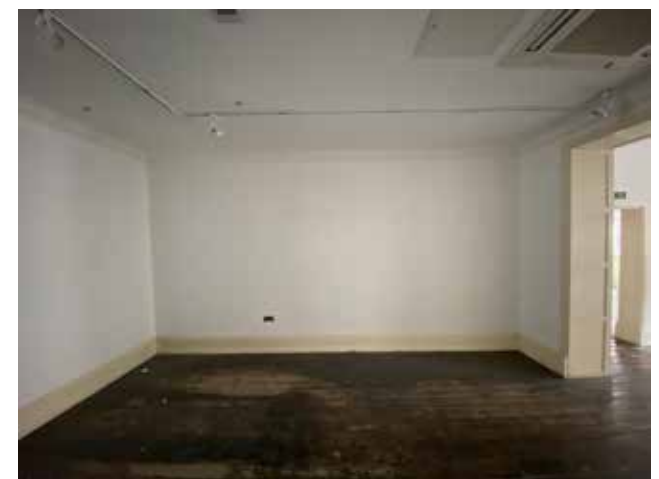
Plate 3.4.89 F.03 view to east partition wall
