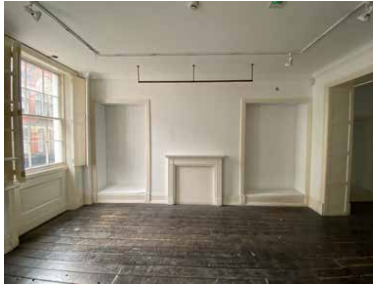
Plate 3.4.77 F.02 view to west outer wall
