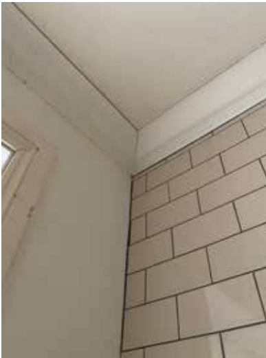
Plate 3.4.101 F.04 Cornice detail over glazed tiles
