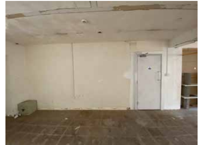
Plate 3.4.151 S.03 view to partition with stairwell
