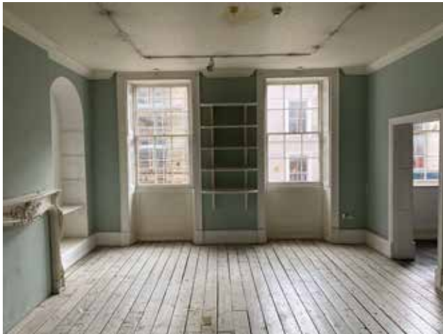
Plate 3.4.105 F.05 view to south outer wall
