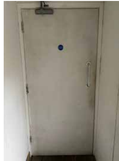
Plate 3.4.103 rear side of door in F.04
