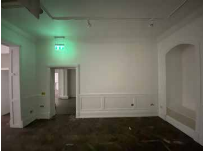
Plate 3.4.42 G.04 View to west partition wall
