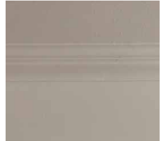
Plate 3.4.20 G.02 Cornice detailing, with evident oin
