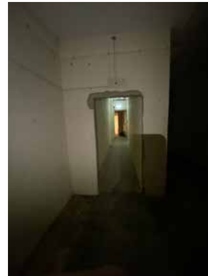
Plate 3.4.192 Basement room B.03, modern access ramp
