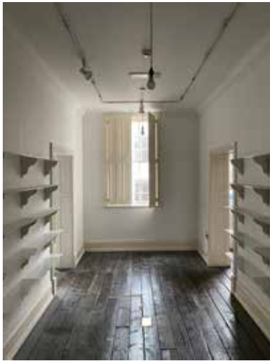
Plate 3.4.61 F.01 view to south outer wall
