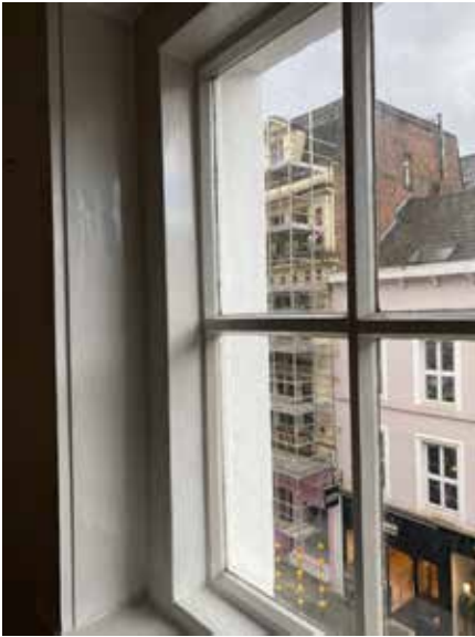
Plate 3.4.146 S.02 Front elevation casement reveal detail
