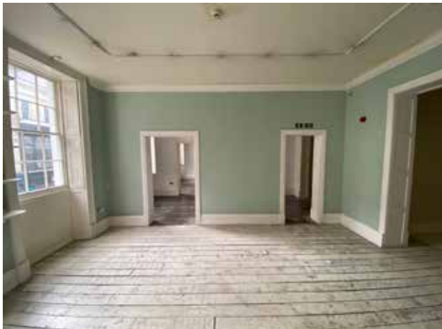
Plate 3.4.108 F.05 view to west partition wall (F.01 beyond)
