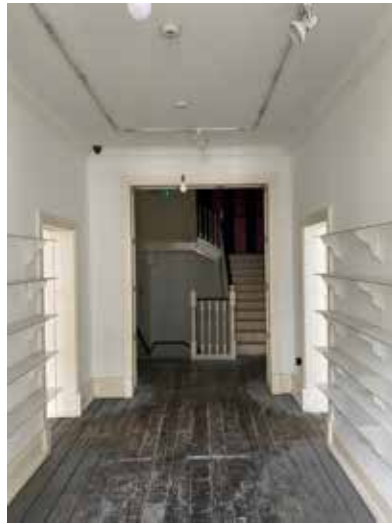
Plate 3.4.62 F.01 View north to stairwell
