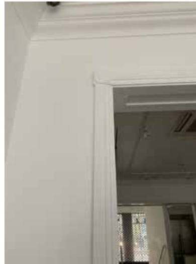
Plate 3.4.22 G.02 Architrave detailing around opening to G.03
