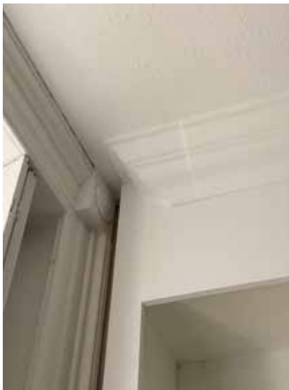
Plate 3.4.56 G.05 Cornice and window architrave detailing, also shown is modern retail shelving to west partition wall
