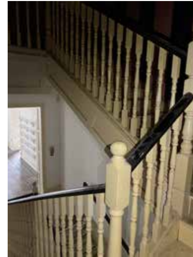
Plate 3.4.172 balustrade turn from first to second floor
