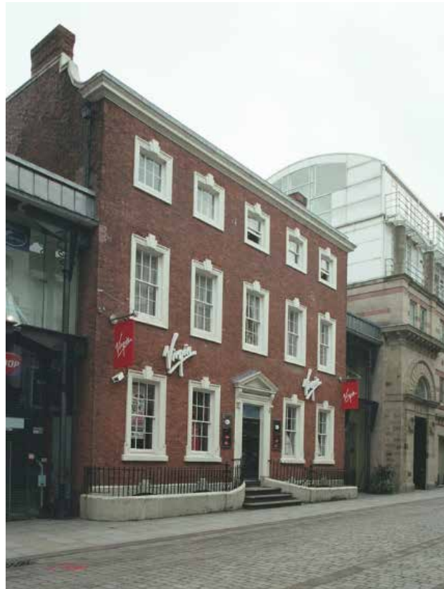
2.39 King Street elevation with Virgin signage, 2004 (Historic England)
