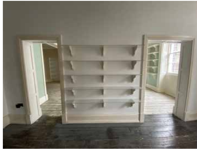
Plate 3.4.63 F.01 view to east partition wall
