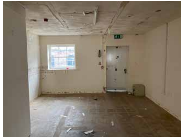
Plate 3.4.150 S.03 view to north outer wall
