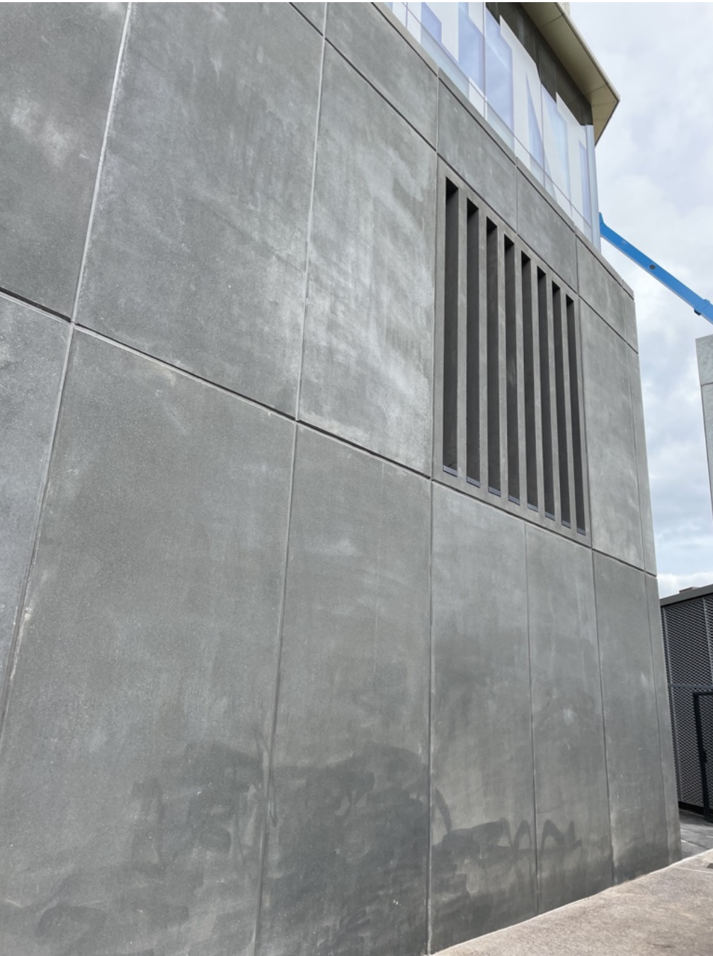
AS BUILT IMAGE 01 - LEVEL 01, WEST ELEVATION
