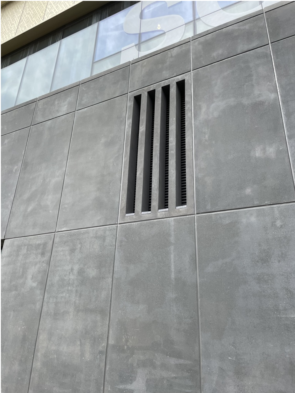
AS BUILT IMAGE 02 - LEVEL 01, WEST ELEVATION
