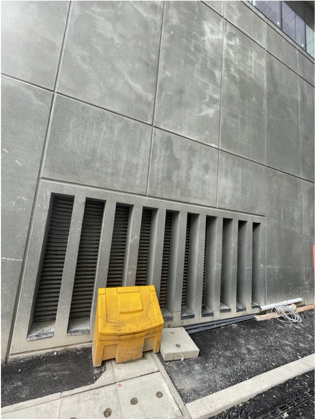
AS BUILT IMAGE 03 - LEVEL 00, EAST ELEVATION
