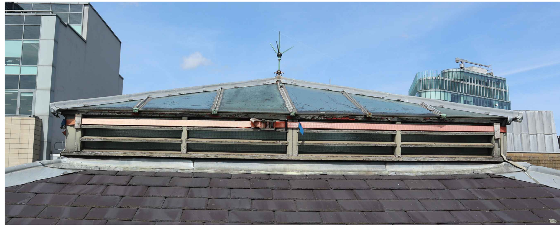
EXISTING ROOF LANTERN PHOTOGRAPH
