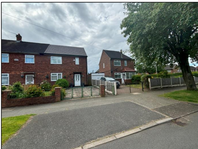
Figure 1. View from Swanage Avenue
