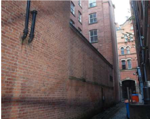
1. Alleyway wall currently demolished to be partially reconstructed with similar/reclaimed materials
