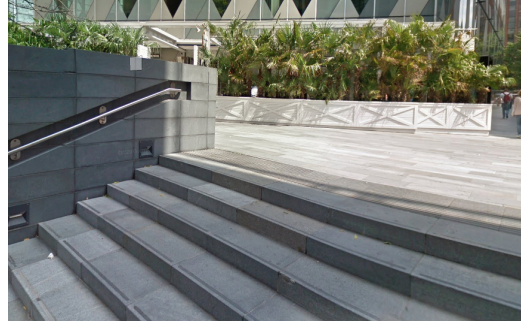
4. Example of stone stair
