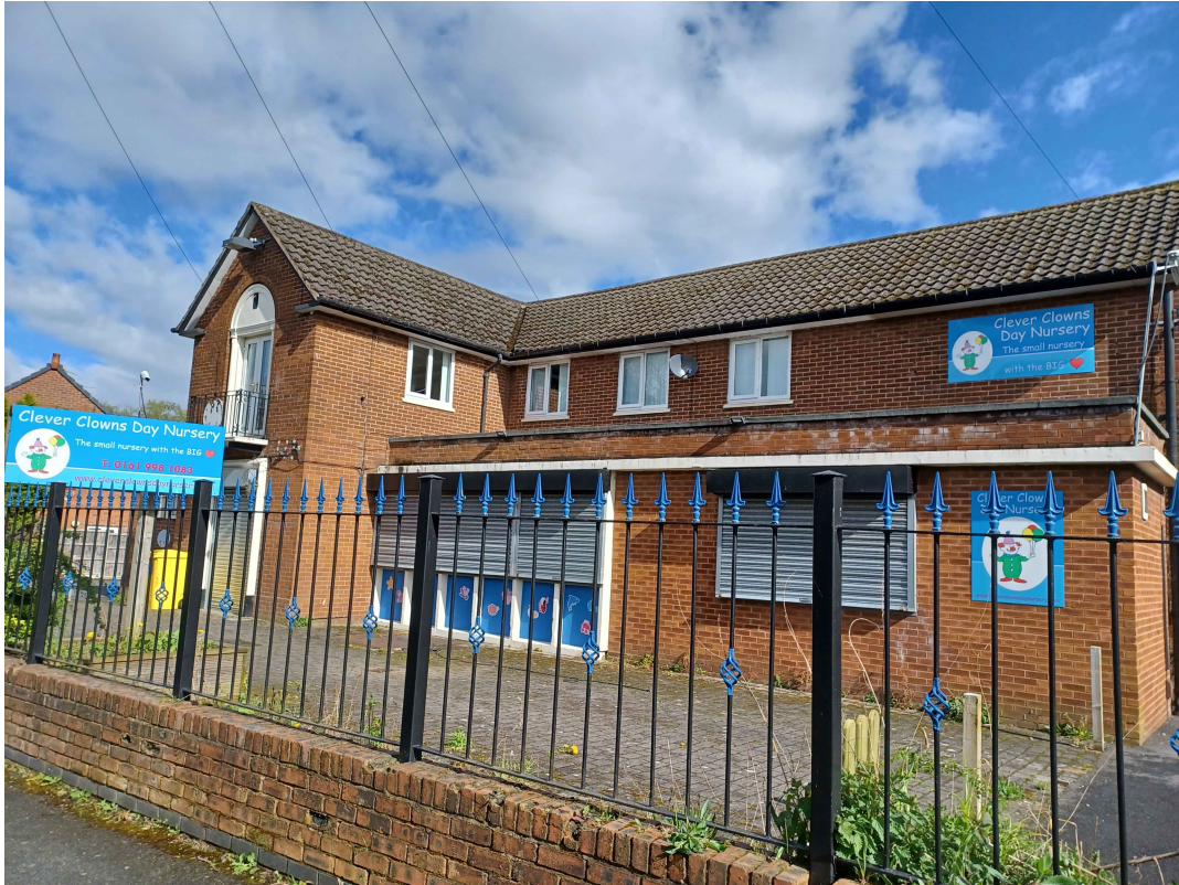
The existing two storey vacant nursery building
