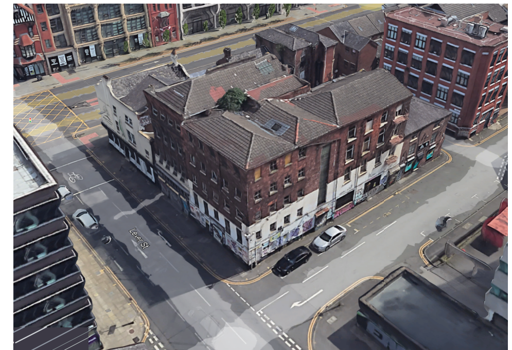
Figure 1.2 Site - North-west corner
