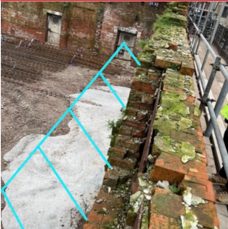
AREA WHERE BAD BRICKS WILL BE PUT - GWS TO CRUSH AND USE IN FOUNDATION BUILD UP.
