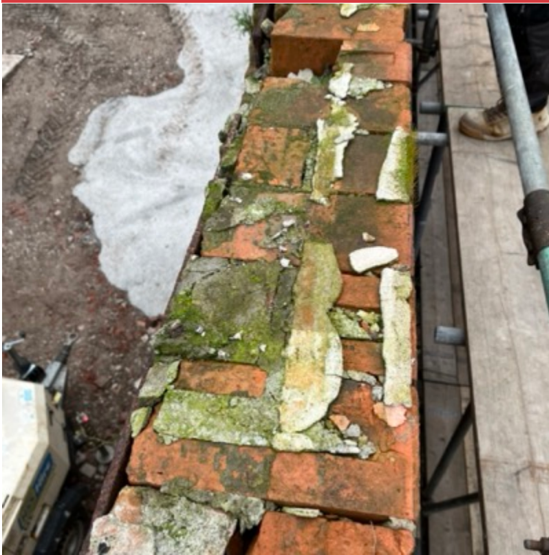
GOULDEN STREET - TOP OF WALL DUE TO COME DOWN
