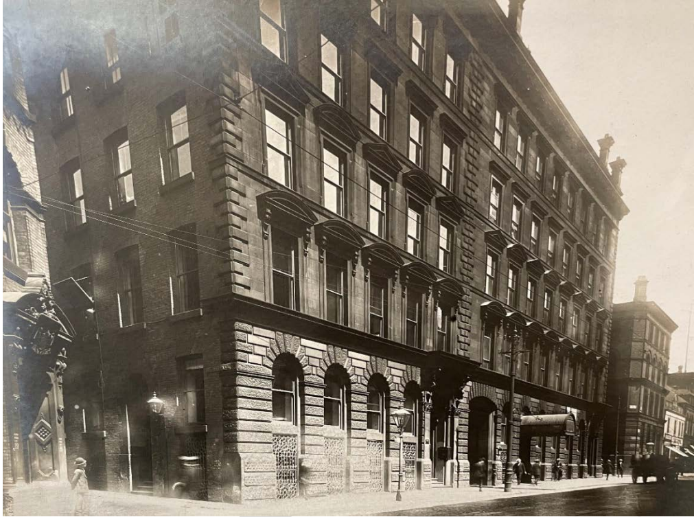
Figure 10 – A photograph looking east along Peter Street towards 37 Peter Street in c1914, showing the now demolished 35 Peter Street to the left, which was also designed by Clegg & Knowles in a matching style to 37. Note the use of a projecting canopy from a ground floor window by this date (Source: Manchester Archives)
