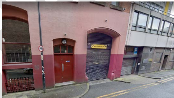
Figure 17: The Bootle Street (north) elevation.
