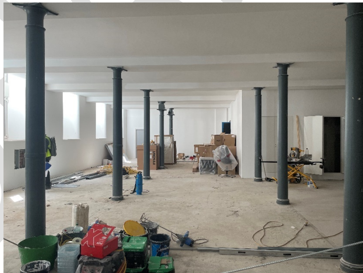
Figure 19: A view looking south through the main room.
