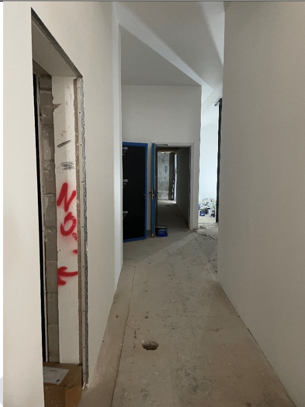
Figure 26: A view looking west across the southern part of the unit, showing the back of house, toilet and kitchen areas.
