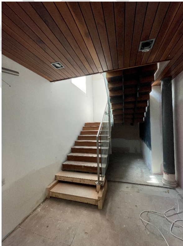
Figure 27: The current, existing modern stairs leading from lower ground floor to ground floor street entrance.
