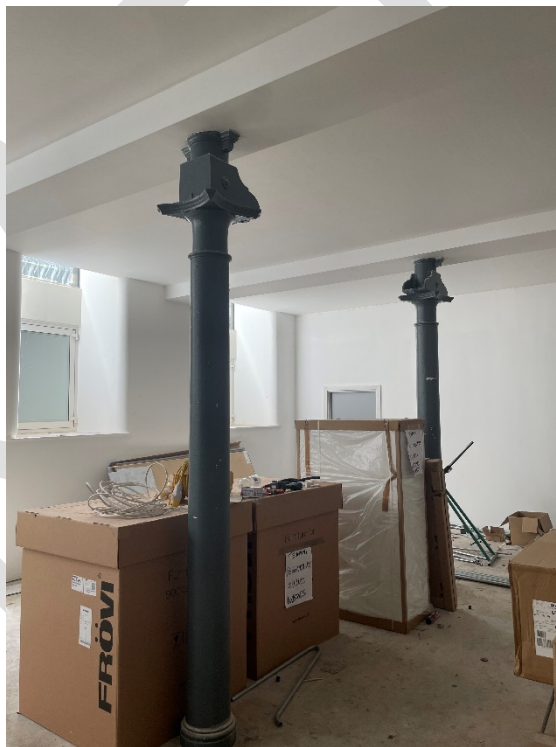
Figure 21: Two columns to the south-east corner of the main room that contain decorative brackets that originals supported the principal staircase.
