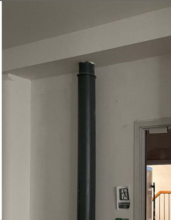
Figure 18: This photo shows the column immediately beneath that shown at ground floor level in Figure 17 above, showing the recently completed fire protection works to the column and beam at lower ground floor level, which has concealed the column capital and moulded beam from view.
