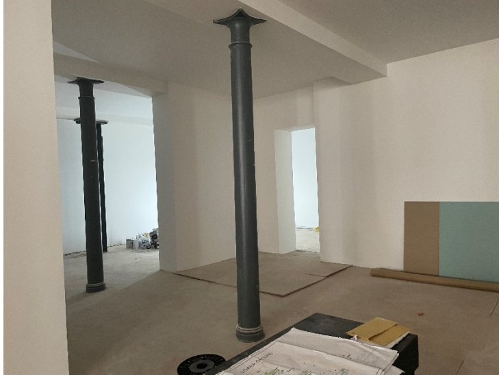
Figure 24: A view looking across the proposed kitchen area.
