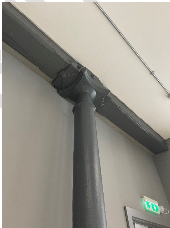
Figure 17: An example of a recently restored original column and moulded timber beam on the ground floor level.
