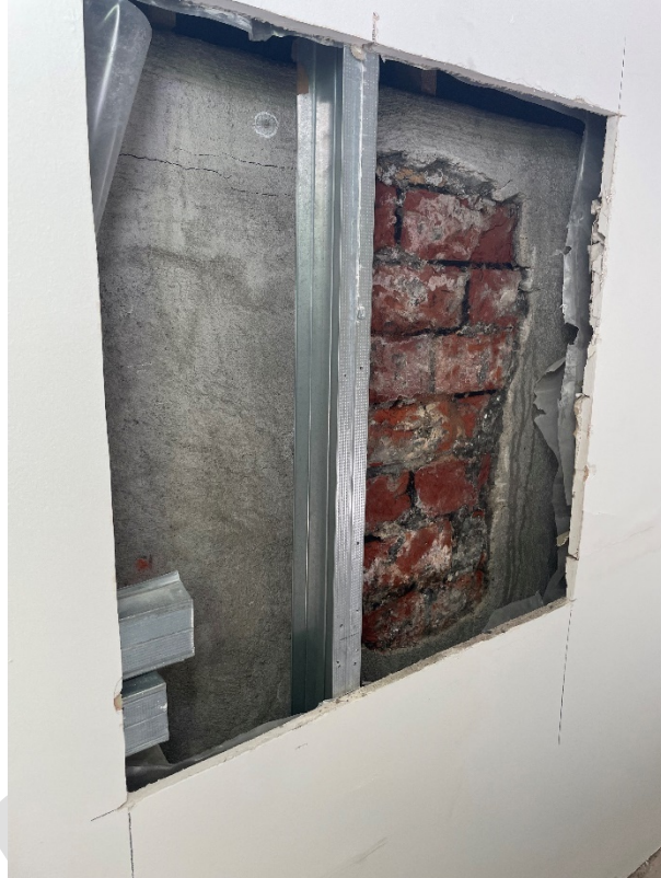
Figure 22: An example of the recent intrusive survey of the tanking system/stud wall to the external walls of the lower ground floor level unit, showing the original brickwork behind.
