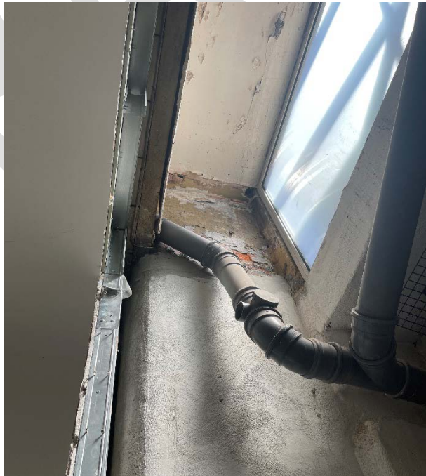
Figure 23: A view looking up into the north-eastern most window opening, showing the original painted brickwork to the top, modern tanking render beneath and modern studwork wall to the left.
