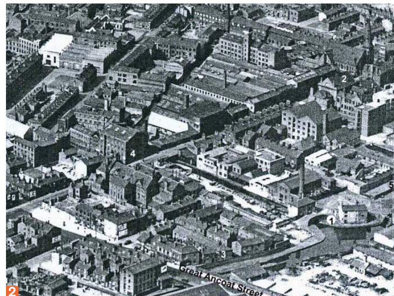
1 Grade II Listed Ancoats Dispensary without scaffolding
