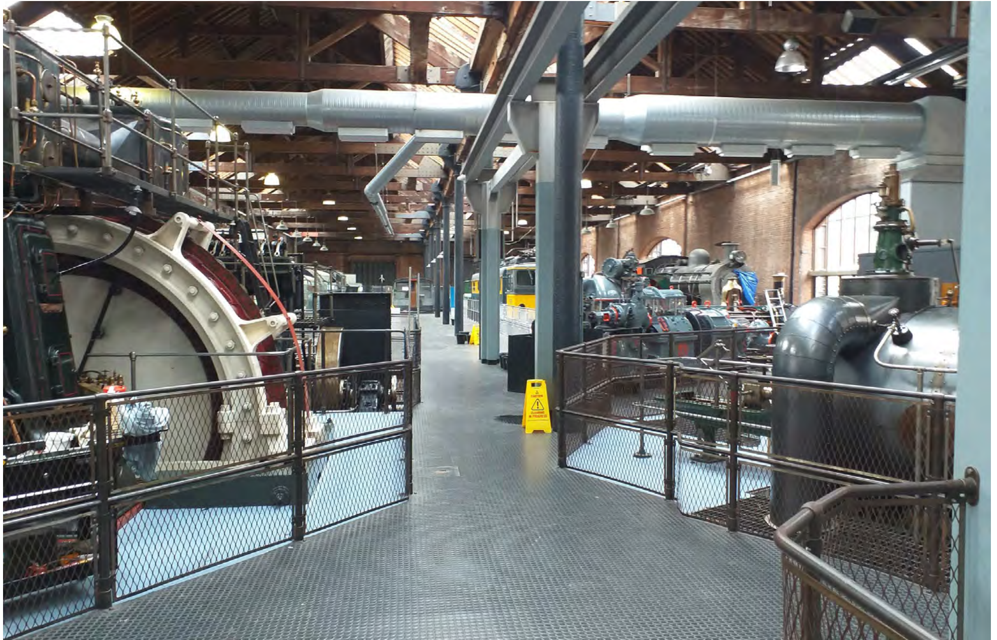
9. The modern raised platform, looking west (Studio Downie)
