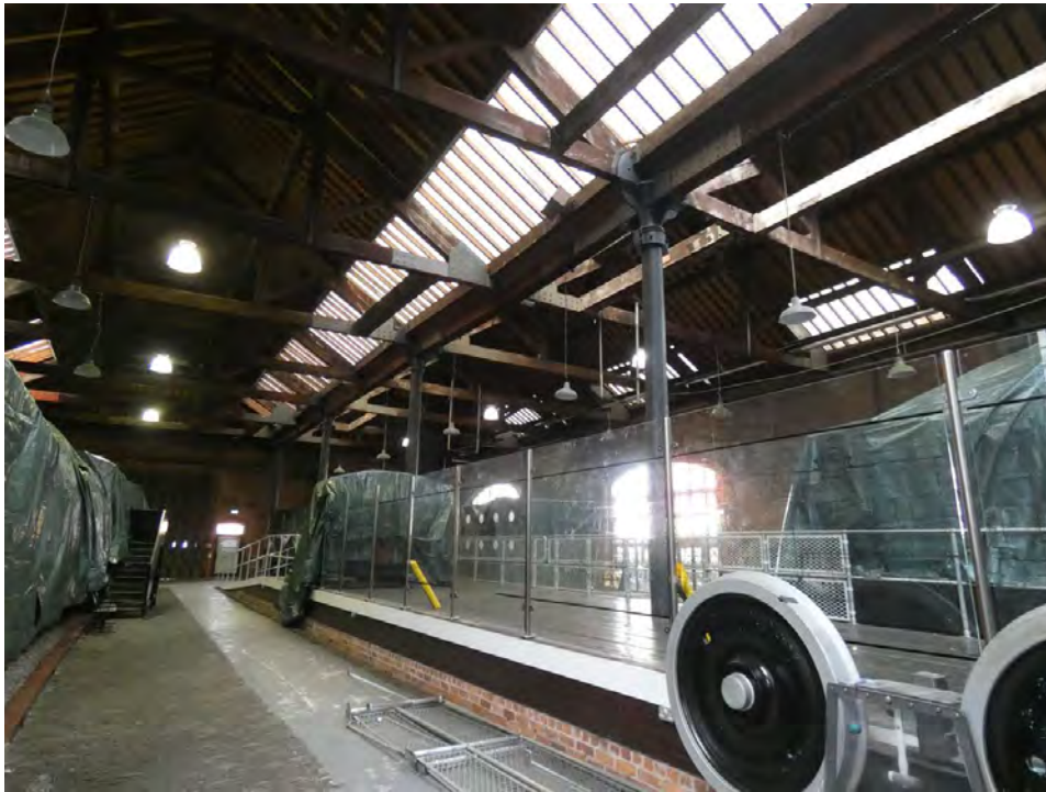
7. Remaining portion of the Central Loading Platform (Insall)
