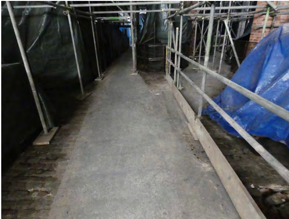
5. Concrete walkway between cobbles (Install)
