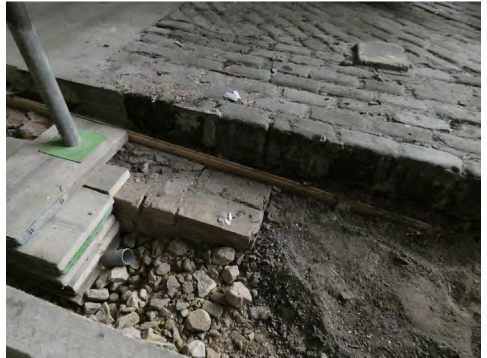
6. Cobbles with modern brick underneath (Install)
