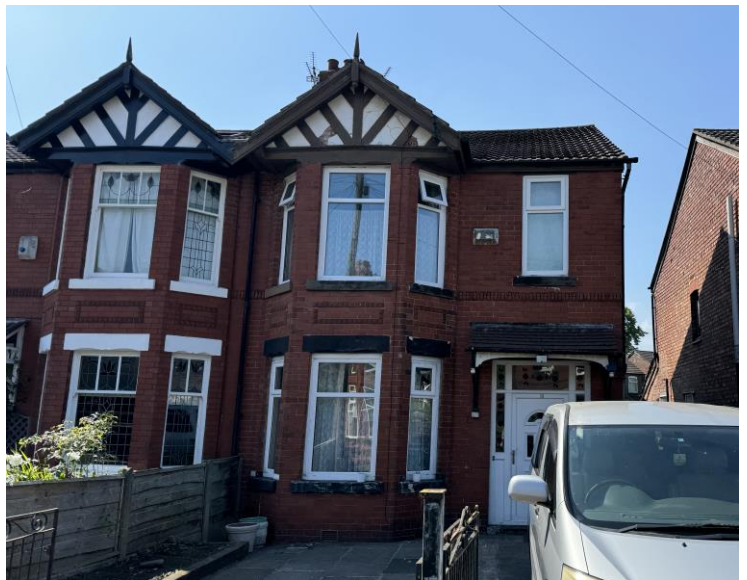
Figure 3. Front view of the property.
