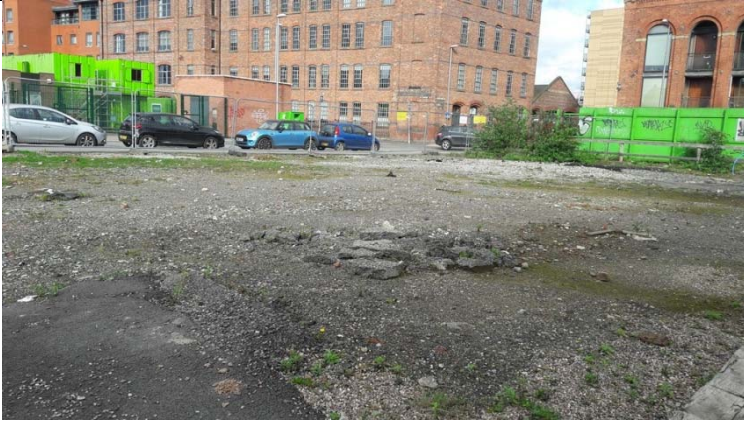
Photograph 2 (P2) Vacant area of land in the north of the site. Hardstood with tarmac in poor condition.
