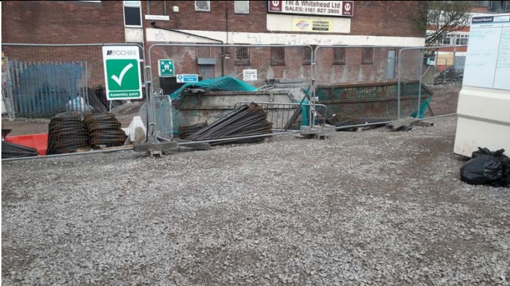
Photograph 4 (P4) Area in south of site also used as a welfare compound and for general waste storage for adjacent construction site.
