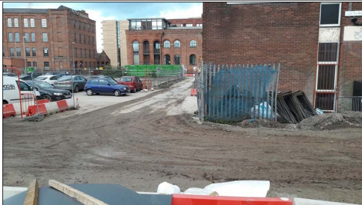
Photograph 1 (P1) View to the north of the site with the adjacent construction site car park visible.
