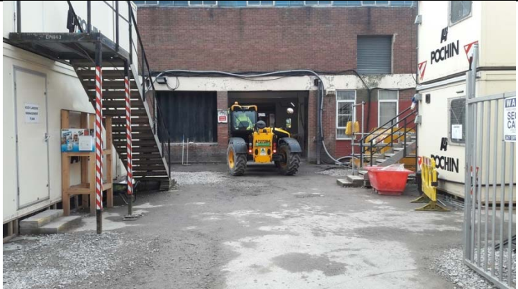
Photograph 3 (P3) Area in the north of the site being used as a contractor's welfare compound. Bunded fuel tank noted in this area.
