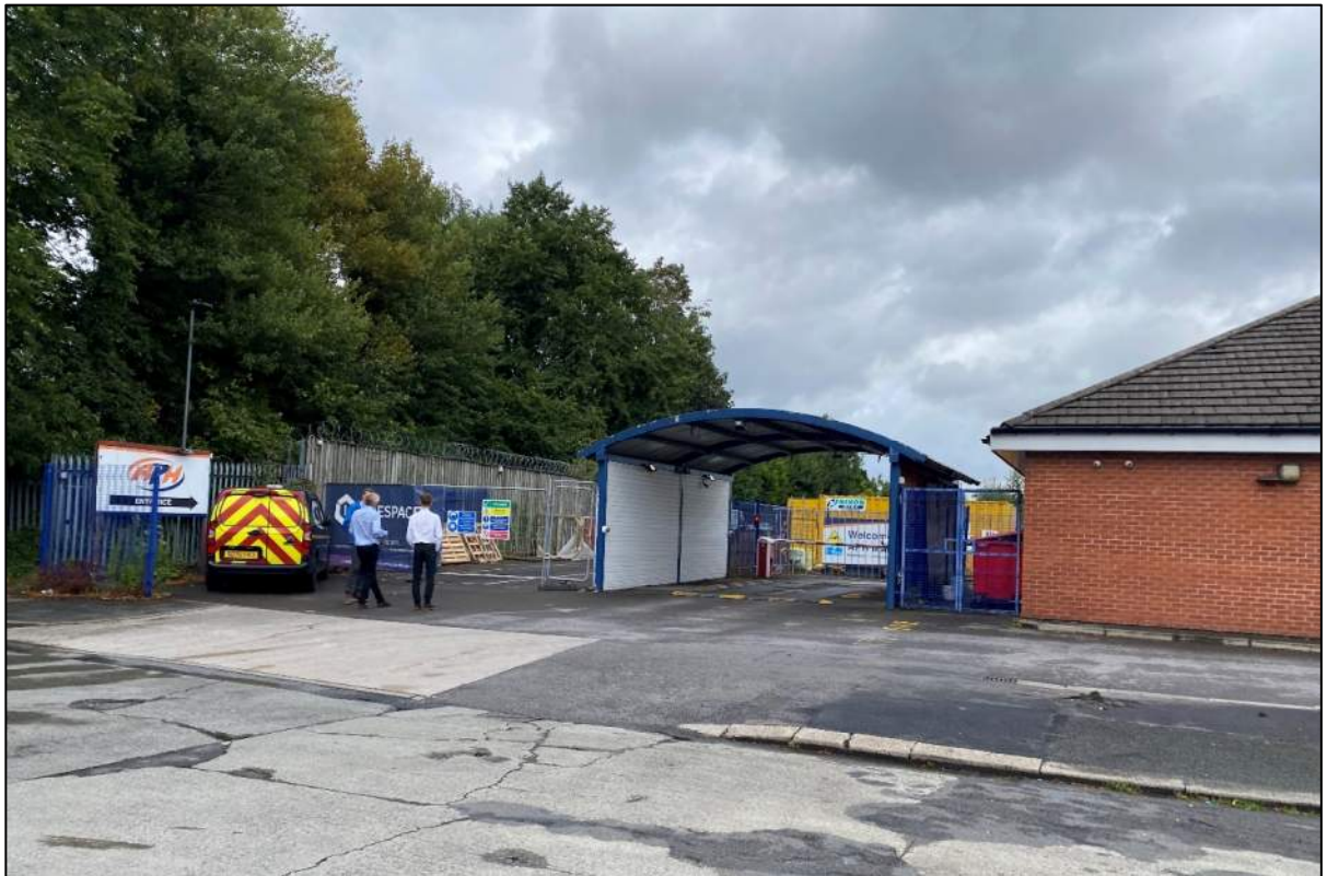
Figure 2.4 – Existing Site Entrance
