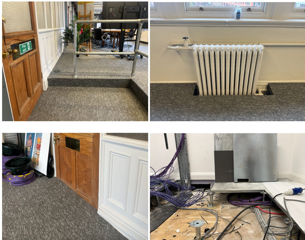
Figs 1, 2 and 3: Modern raised floor within Breakout Room and Sting Room which covers the existing doors, skirting and radiators. Figure 4: Example of raised floor method of construction (from other section of the building).
