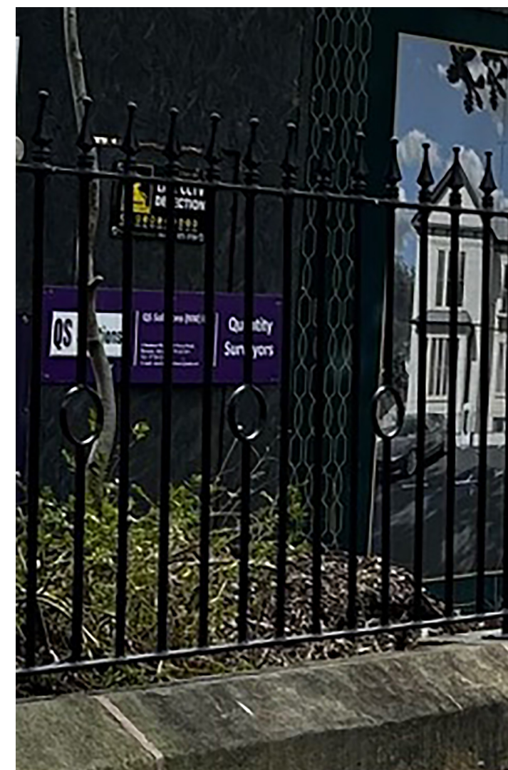
Powder coated steel decorative fencing atop reclaimed stone coping/facing brick low-level wall.
