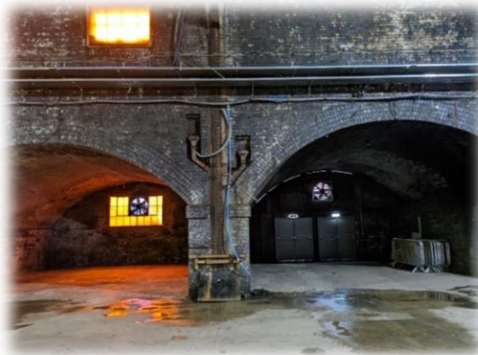
Figure 3 – Concourse bi-directional fans via existing 'Fairfield Street' fenestrations façade.
