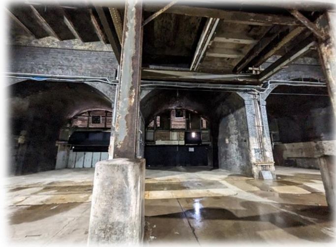
Figure 4 – ‘Depot’ bi-directional fans via existing ‘Fairfield Street’ fenestrations façade.
