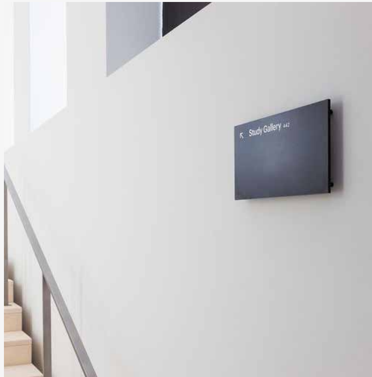
Aluminum sign panel raised off of wall
