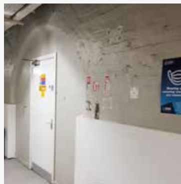
Mixture of painted exposed brick and plaster board
