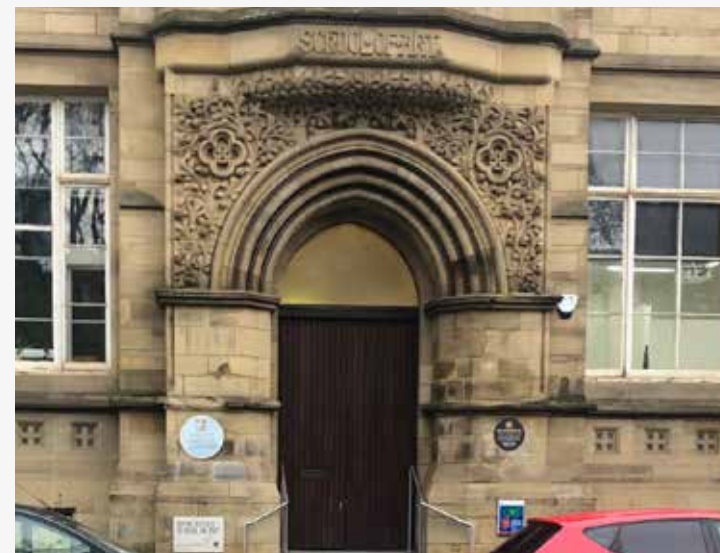
Existing signage at Grosvenor West entrance: 'School of Art' lettering above door, heritage plaques on both sides of the door
