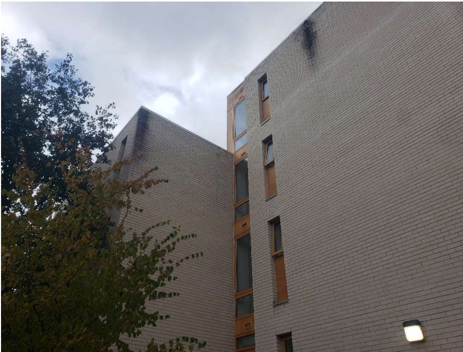
Figure B.6 Gaps where brick slips have broken or become dislodged on B2
