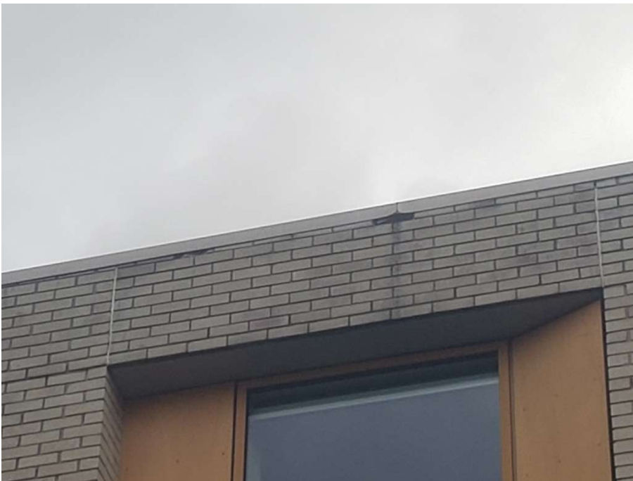
Figure B.6 Gaps where brick slips have broken or become dislodged on B2
