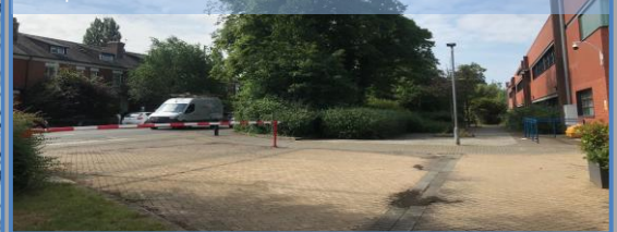
A landscaped pathway separates the eastern elevation of the hospital from Burton Road
