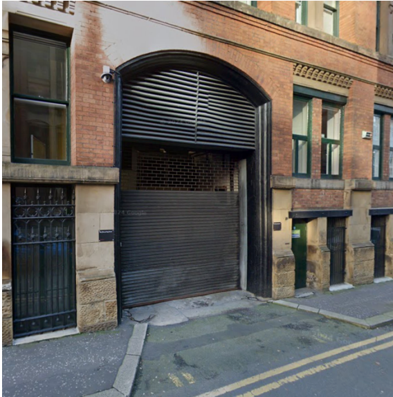
Figure 5: Picture of loading bay on Dickinson Street.
