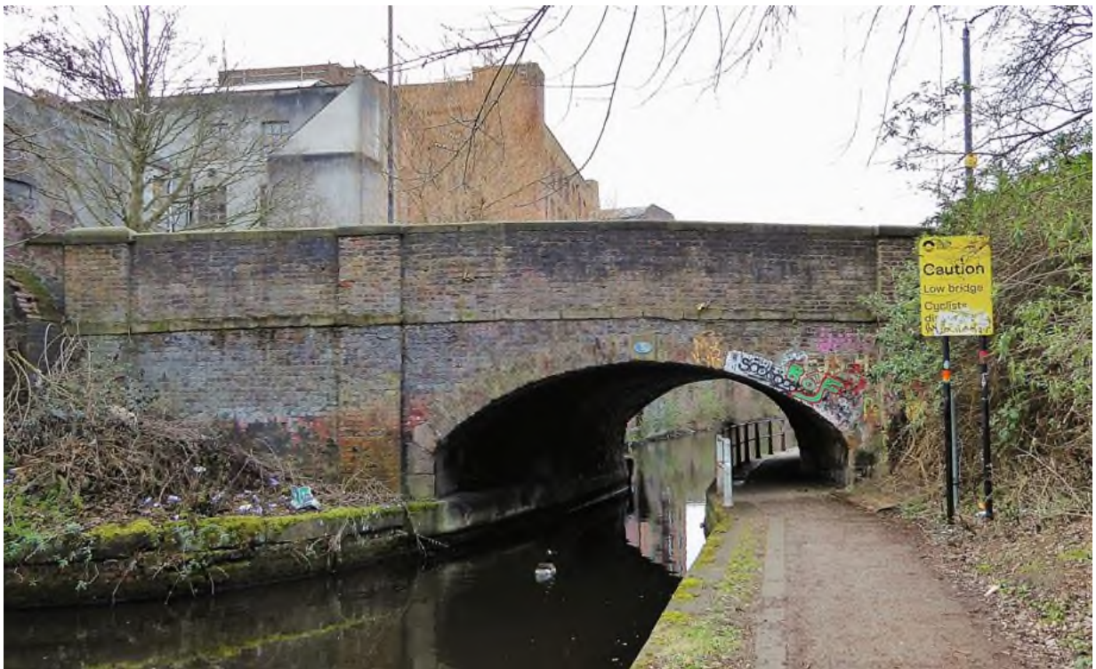
Figure 6-10 Bridge Number 5 Over Ashton Canal (Authors Own)
