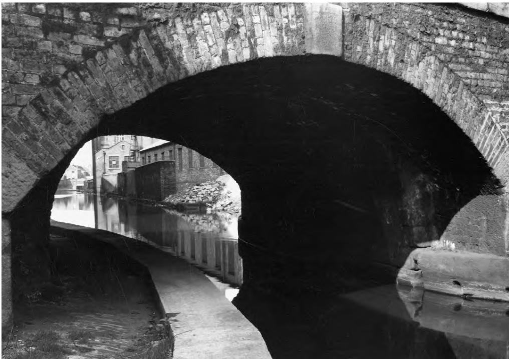
Figure 6-9 Beswick Street bridge in 1962, (Manchester City Council Libraries). Looking north east from the Canal towpath. As shown the area surrounding site is still occupied by industrial uses at this stage, and is densely built along the canal side, however by this stage the canal had become rather unkempt. Many of the industrial buildings would be demolished in the following decade.
