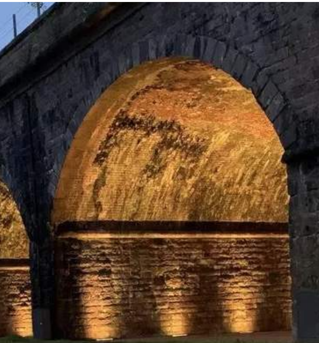
Figure 7: Lighting the surroundings for increased safety
