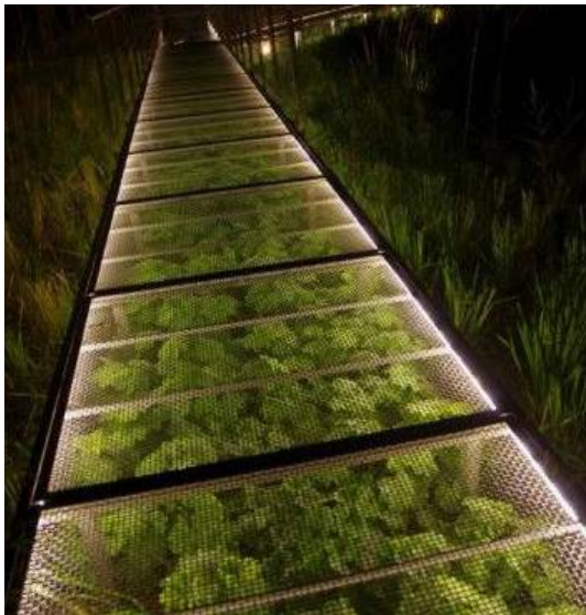
Figure 26: Back-lit mesh walkways
