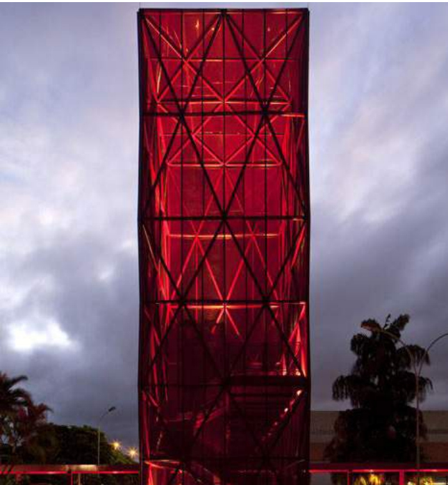
Figure 4: Revealing the structure of the lift and staircase at night
