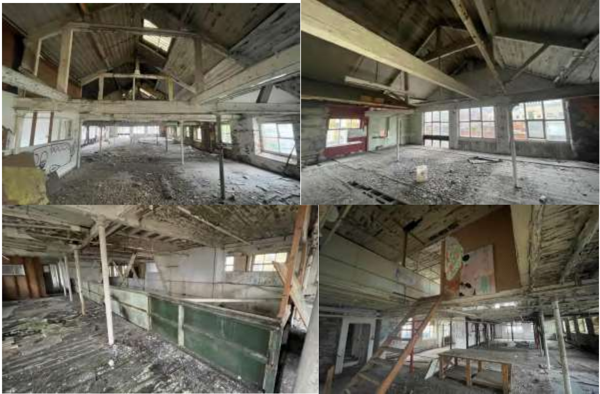
Existing Interior Images
