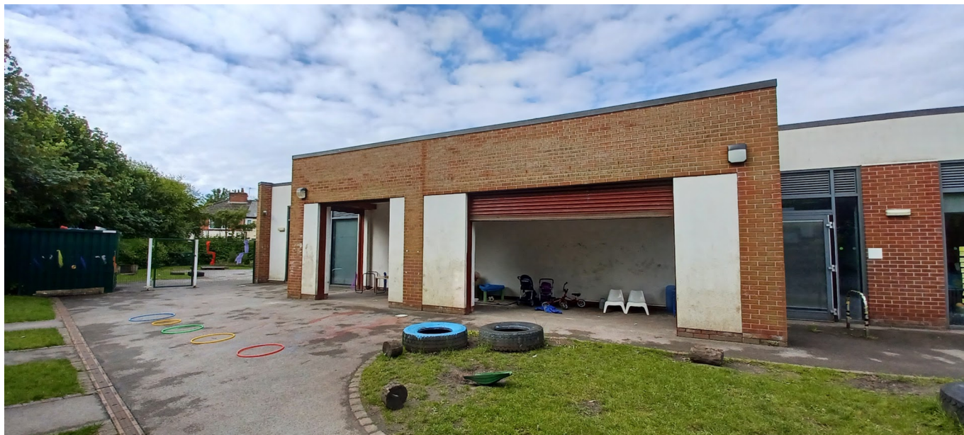
Figure 1. Existing covered play area.
