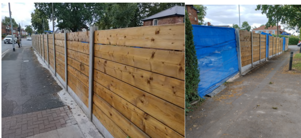
Fig.2 – Views of fencing erected to Old Hall Lane Boundary
