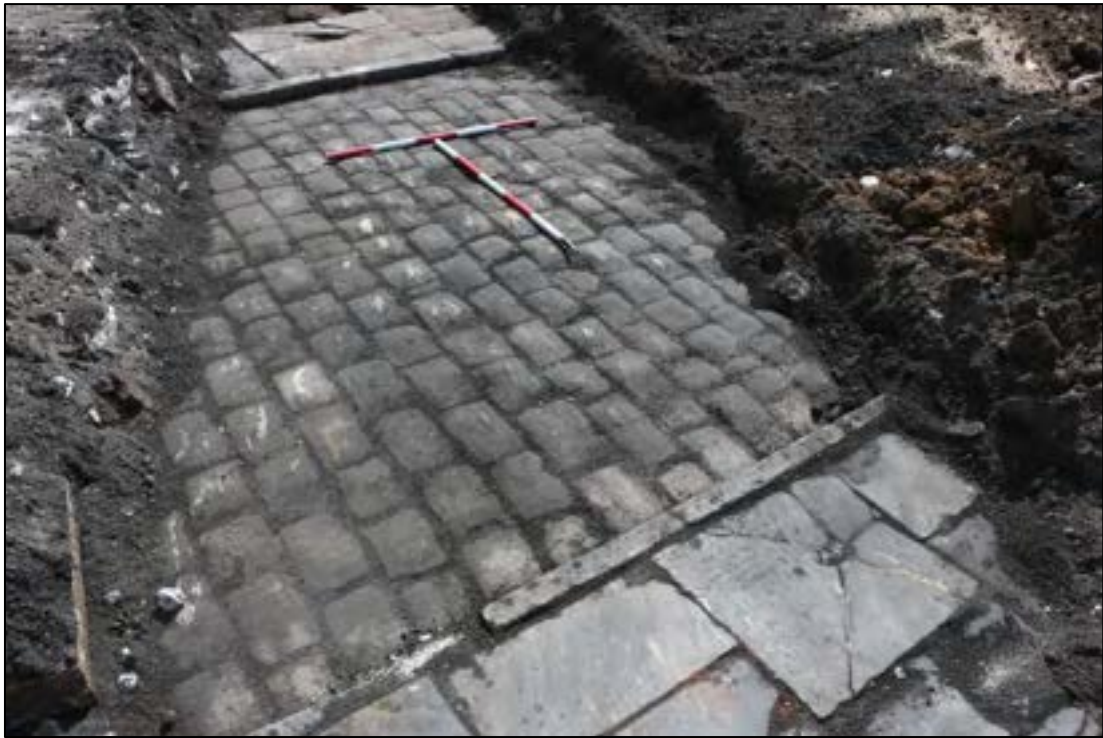
Plate 19: Shot of cobbled road surface [1204] and pavements [1203] in Trench 6, looking south-east. Scales = 2 x 1m.
