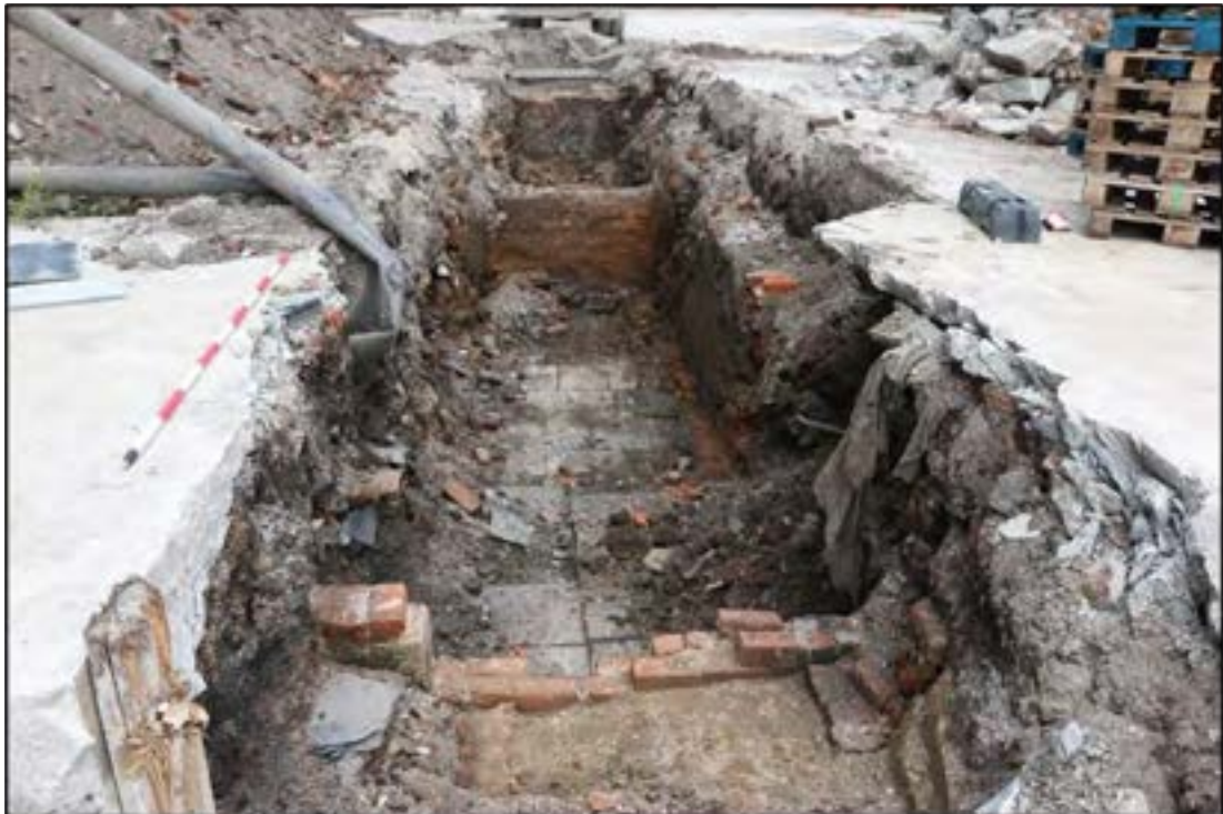
Plate 9: General shot of Trench 3 showing 19 th -century house remains, looking north-east.
