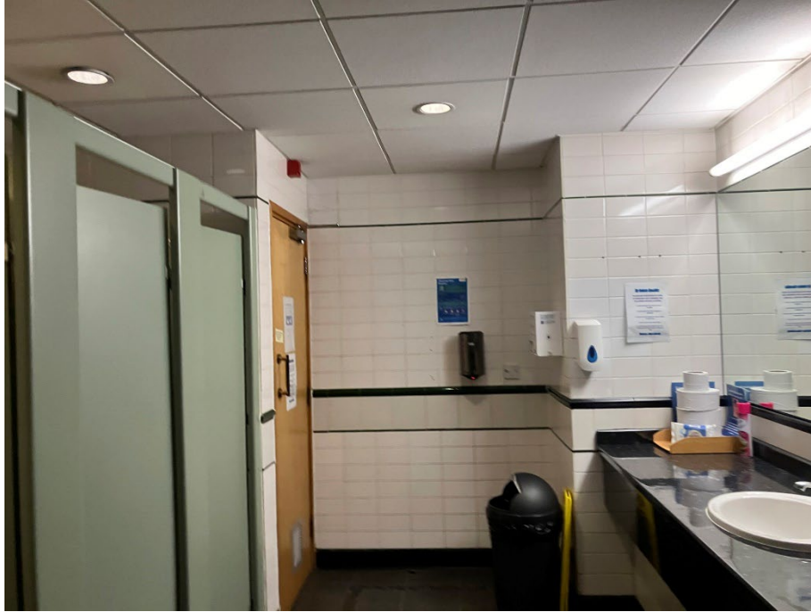
Figure 21: A typical view of one of the toilets seen across both office units, showing modern fit-out/tiling etc.
