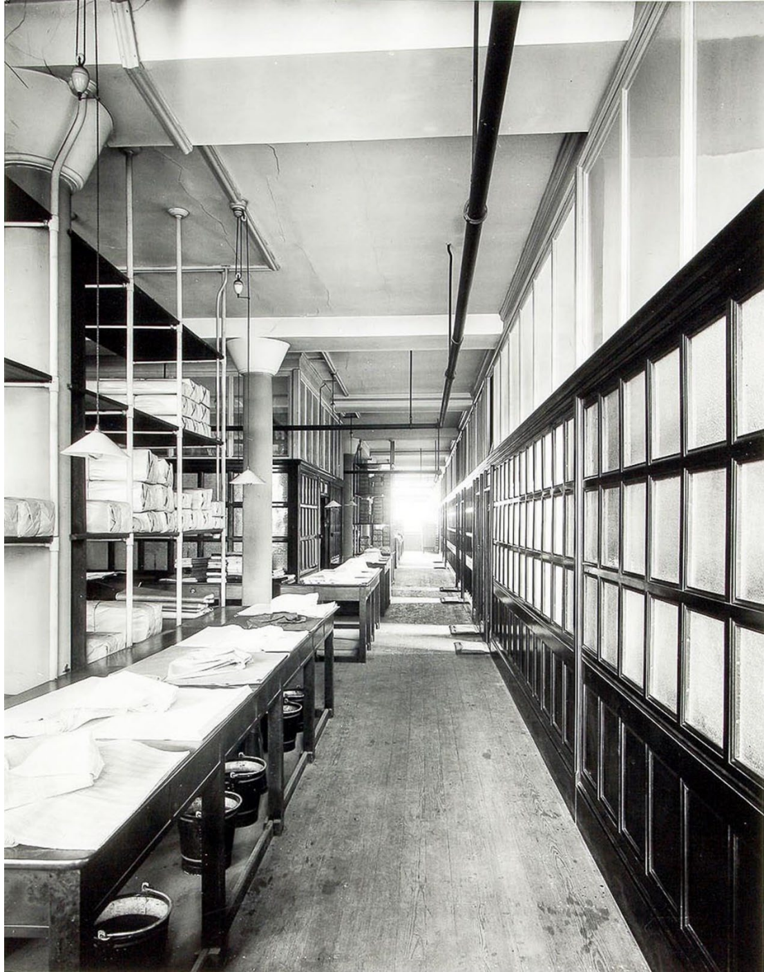
Figure 6: This photograph represents one of the warehouse spaces on the first floor of the building, and illustrates the type of circular, reinforced concrete column that survives today. (Source: Historic England Archive)
