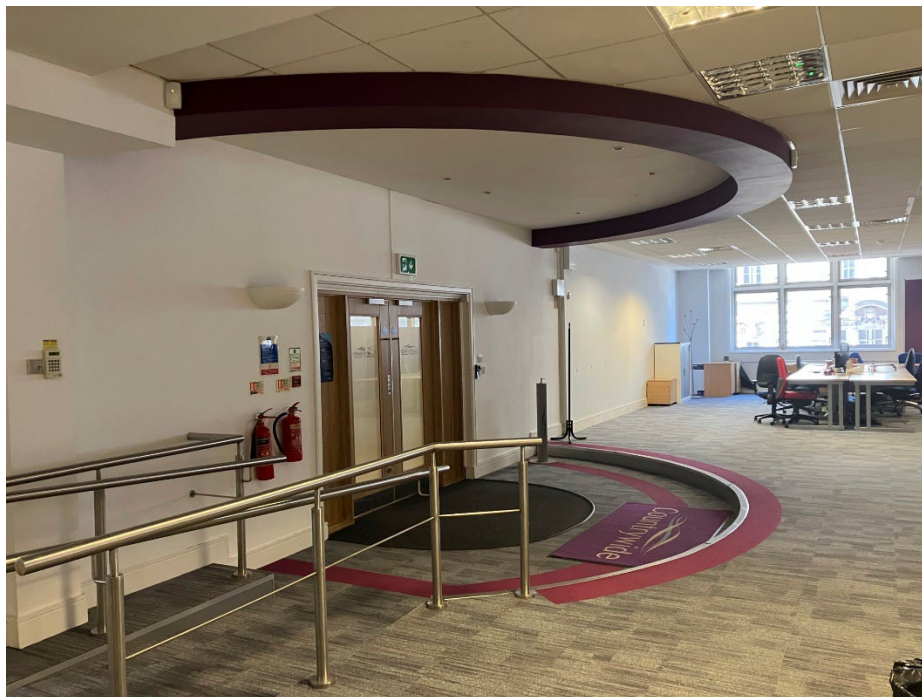
Figure 16: Looking towards the principal second floor entrance into the Countrywide unit in Churchgate House from within the unit, showing the modern raised access floor/railed ramp and dropped ceiling.
