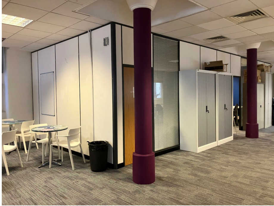
Figure 19: An example of a shallower dropped ceiling which partially obstructs views of the original columns in Churchgate House.
