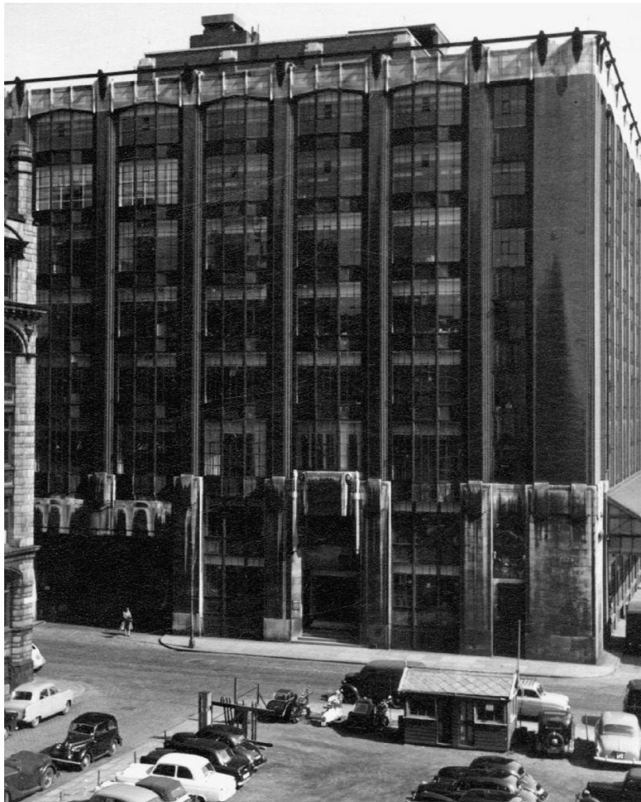
Figure 7: The northern elevation of Lee House in the 1950s (Source: Manchester Archives)
