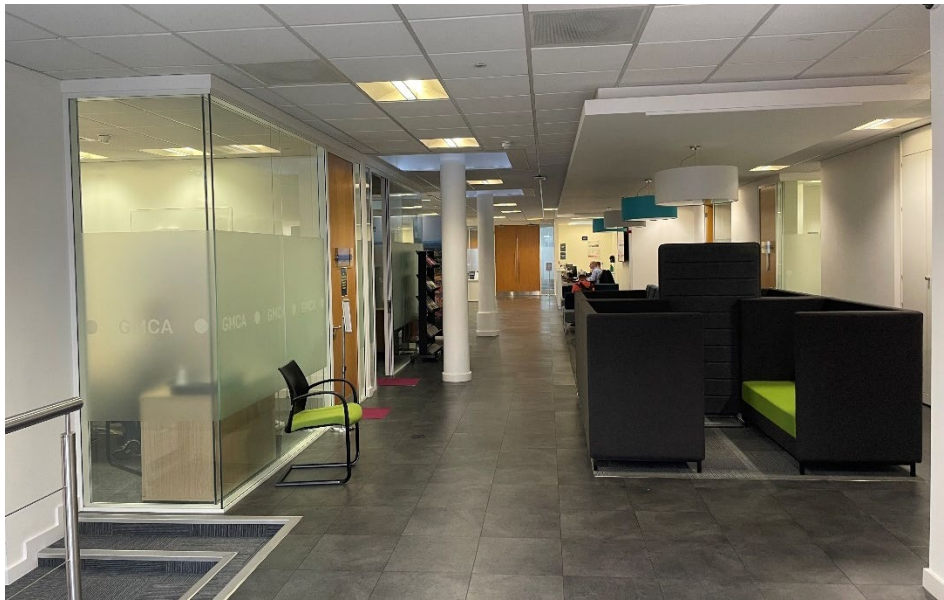
Figure 10: Looking east across the first floor level demise of the unit (Chuchgate House) from its central wing, showing the modern floor coverings, dropped ceiling, raised access floor, office enclosures, skirtings and lighting.
