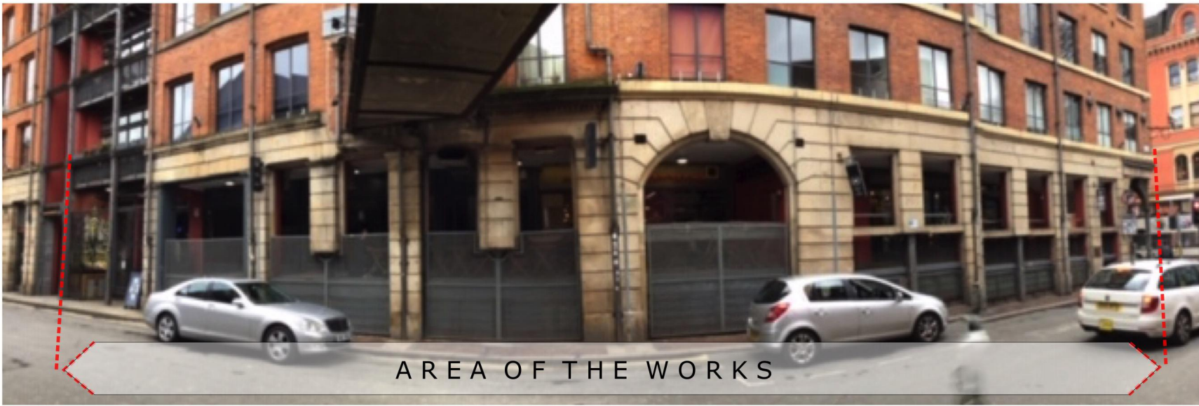
Photograph of the Existing Facade
