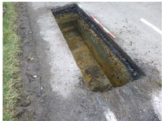
Example of how to photograph an open cut trench excavation. Suggested title 'Trench 1 looking north east'
