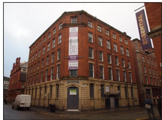
Figure 3: Mindel House (prior to works starting and installation of scaffolding).
