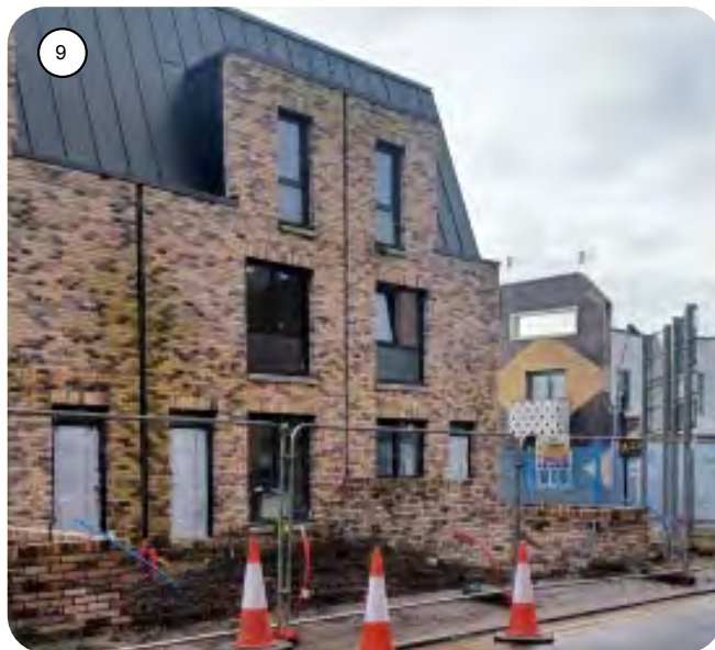
Development under construction in Miles Platting
