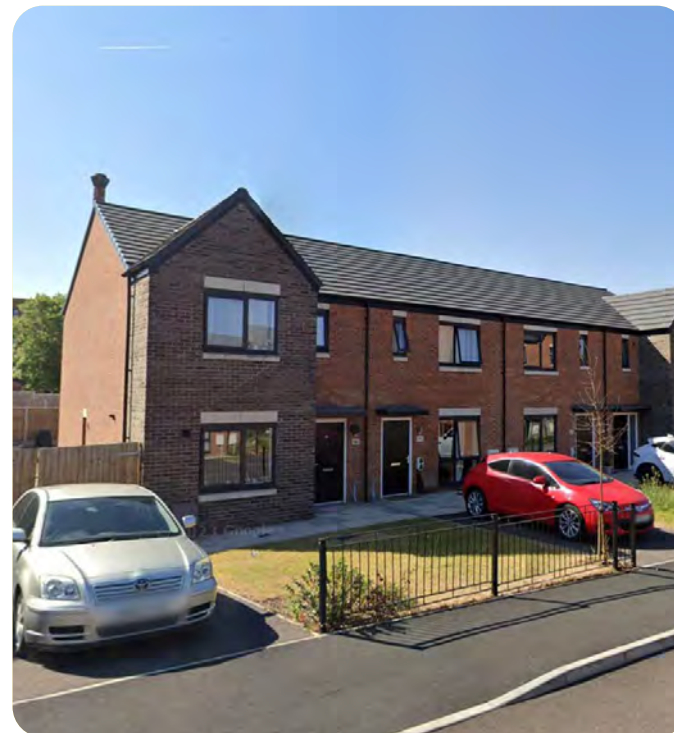
Stone sills Winstanley Road
