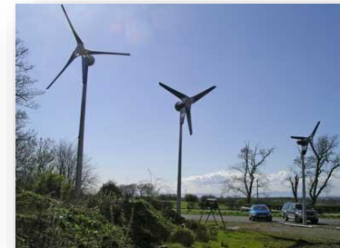
Wind Turbine Installation
