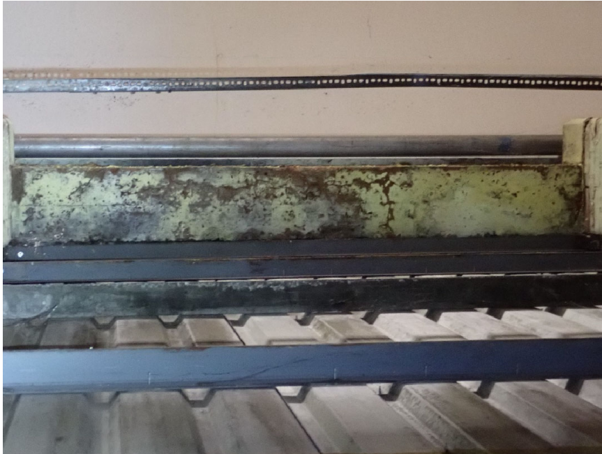
Photo 25. Minor longitudinal cracking to soffit of window 5 internal lintel
