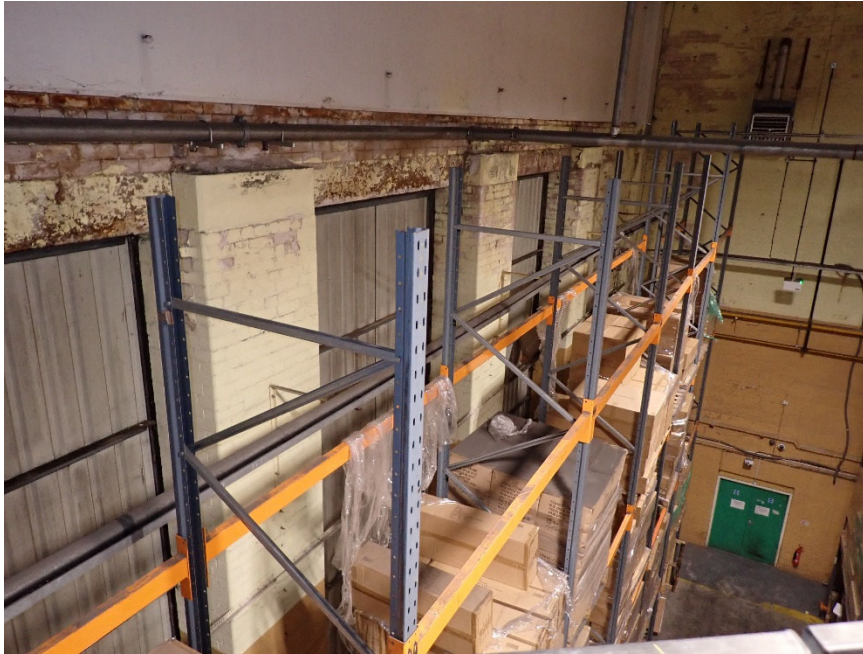
Photo 22. High-bay racking to internal face of north-west elevation
