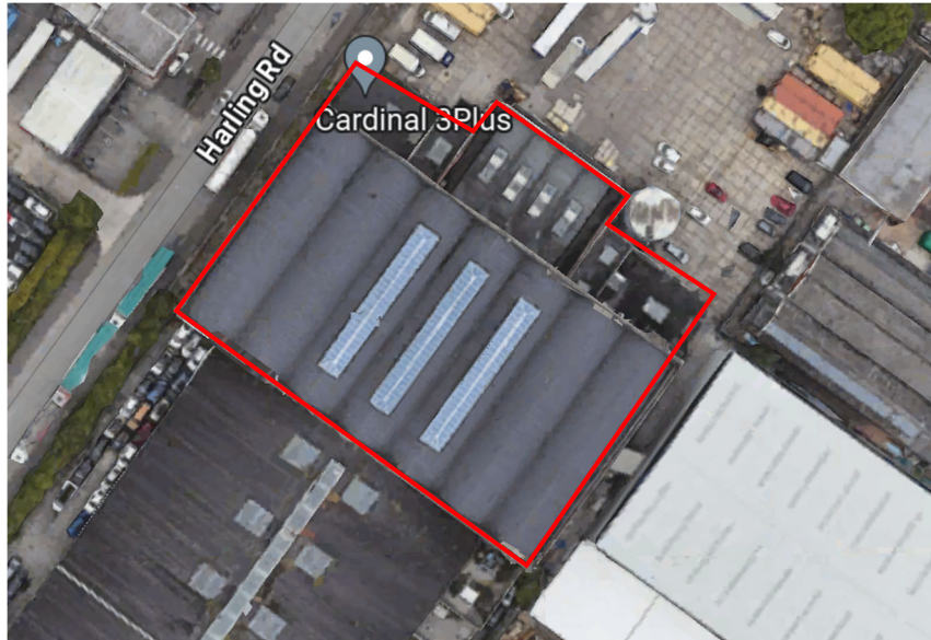
Photo 1. Aerial view of survey area
