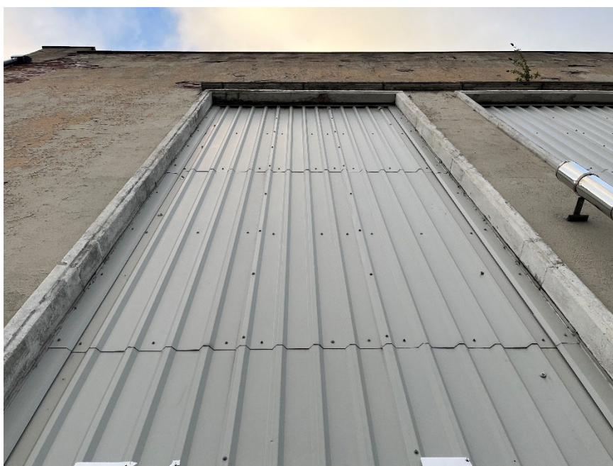
Photo 3. Typical window detail with profiled surround and head
