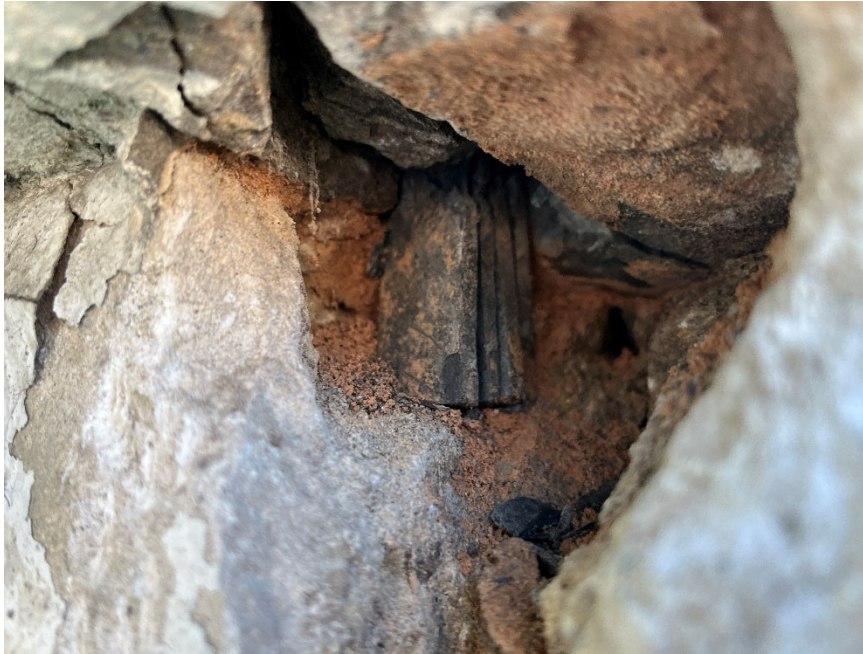
Photo 16. Slate pins between adjacent window surround panels
