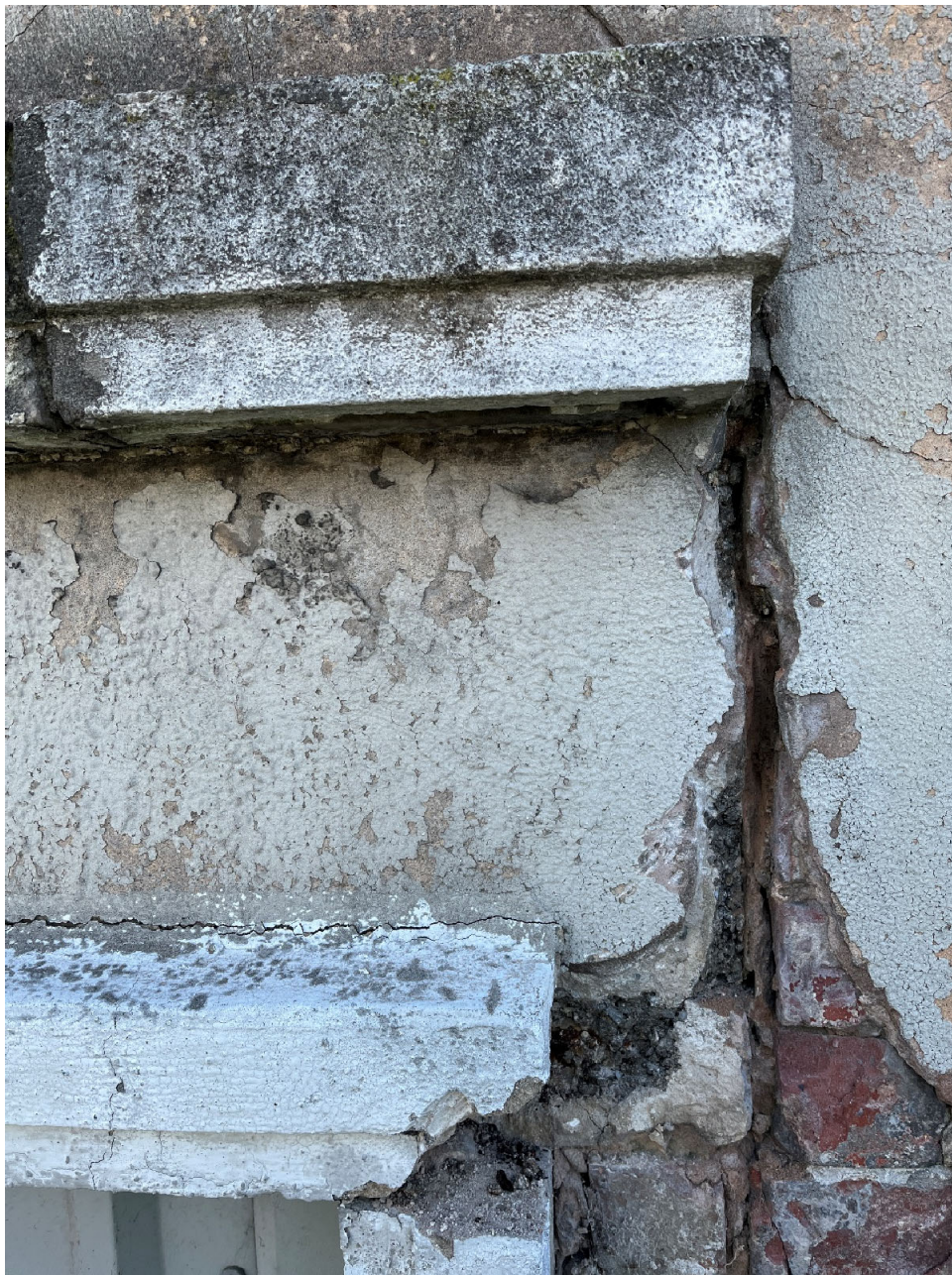
Photo 5. Top right-hand corner of window 8 showing structural arrangement
