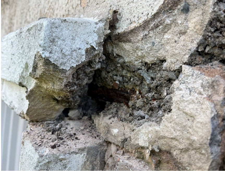
Photo 6. Integral window head and lintel
