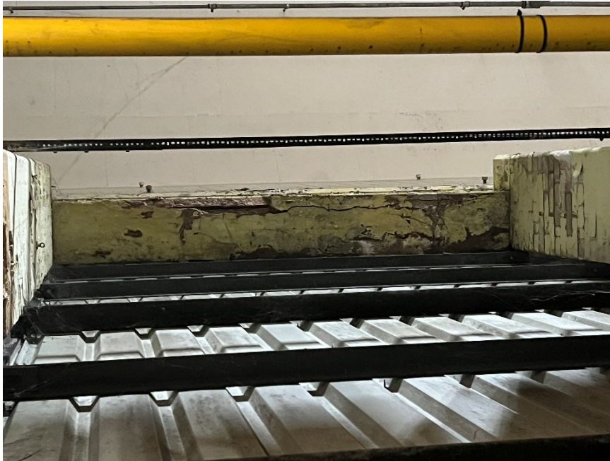
Photo 23. Underside of internal lintel to window 8
