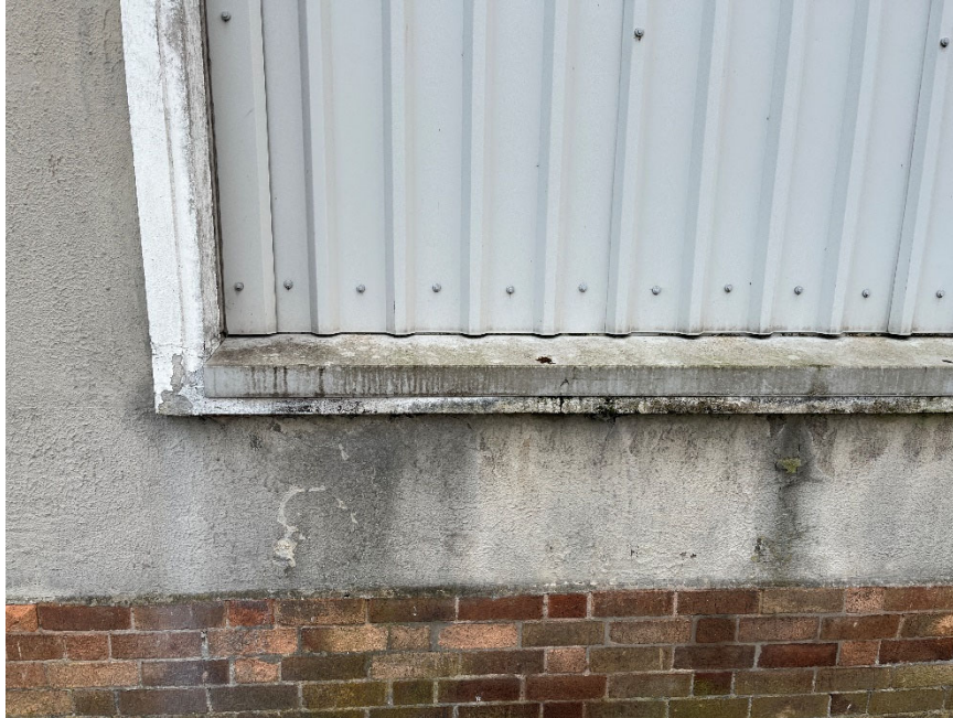
Photo 4. Typical window cill with pressed-metal flashing
