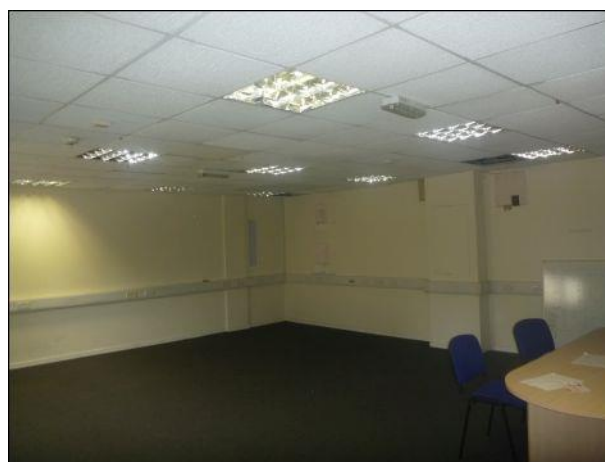
Photo 16: Building 2, upper floor of two-storey section, showing suspending ceiling
