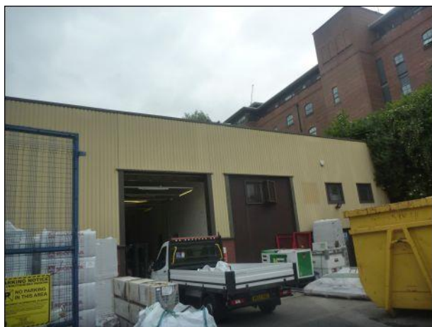
Photo 13: Building 2, western elevation
