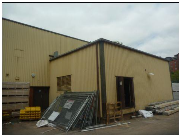
Photo 7: Building 1, eastern elevation, northern end
