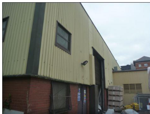
Photo 6: Building 1, eastern elevation, southern end
