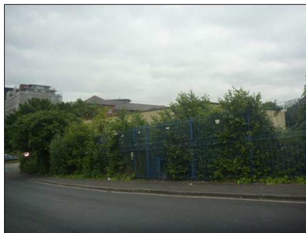
Photo 8: Building 1, western elevation
