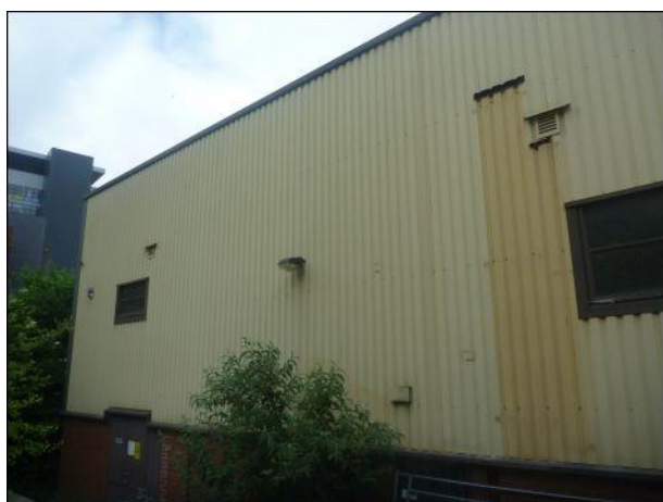
Photo 9: Building 1, southern elevation
