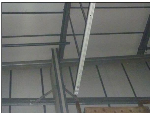
Photo 11: Building 1, internal area, showing underside of roof
