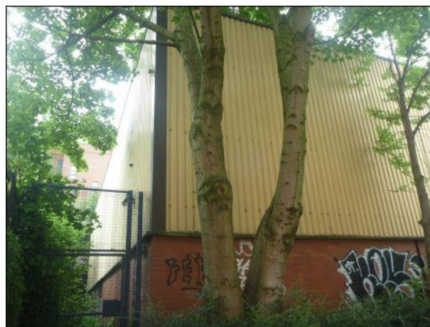
Photo 14: Building 2, eastern elevation
