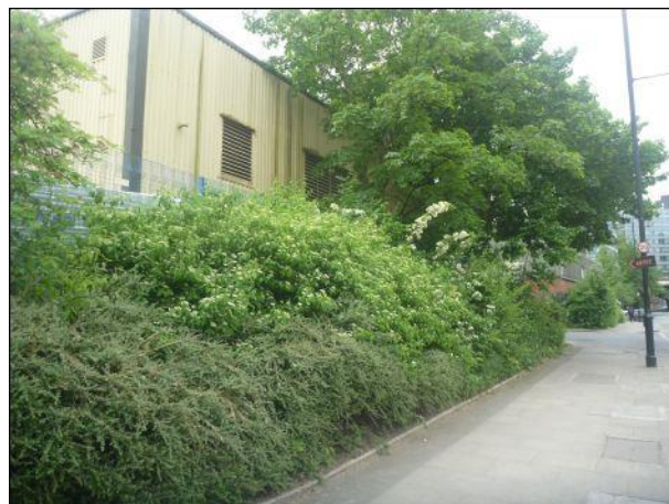
Photo 2: Ornamental shrubs and trees, and northern elevation of Building 1
