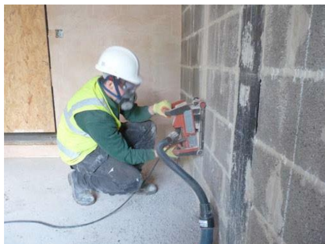
Figure 4 Wall chasing using on-tool extraction
