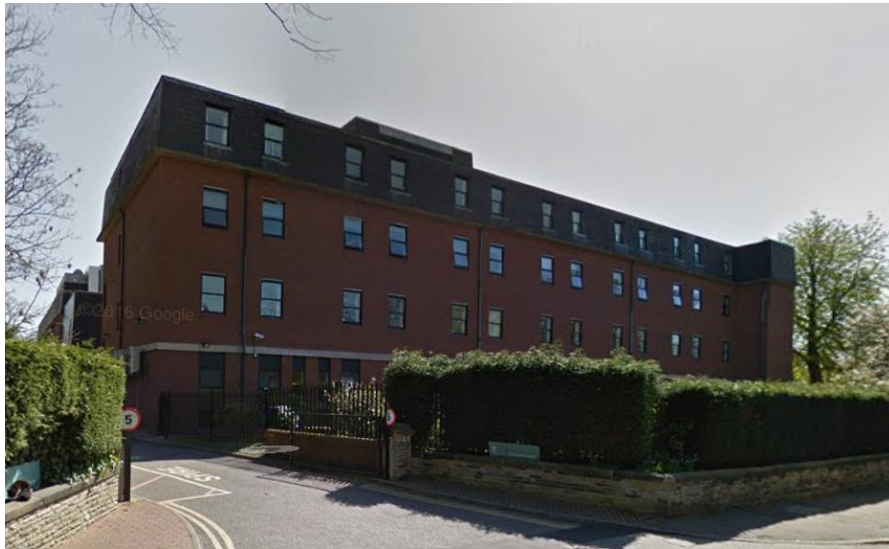
Figure 9. Google Streetview Image of Former Hospital Prior to Demolition circa 2016
