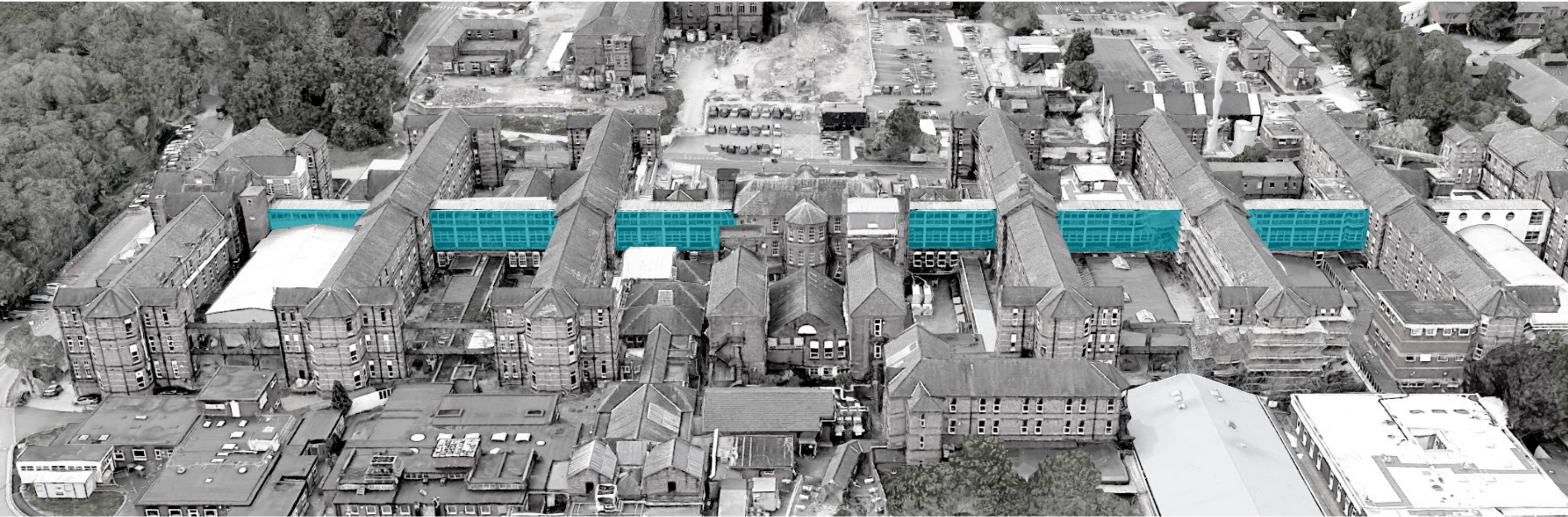
Figure 2: Aerial View of the North Facing Elevation of the NMGH Hospital Site
