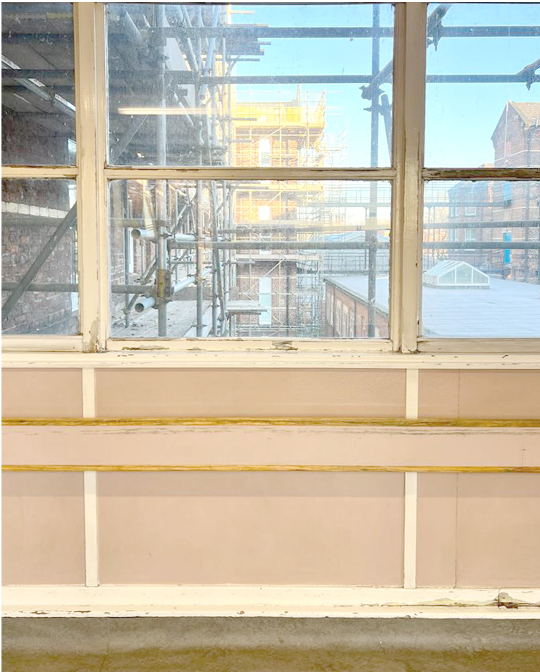
Figure 6: Image displaying internal condition of Corridor Link cladding
