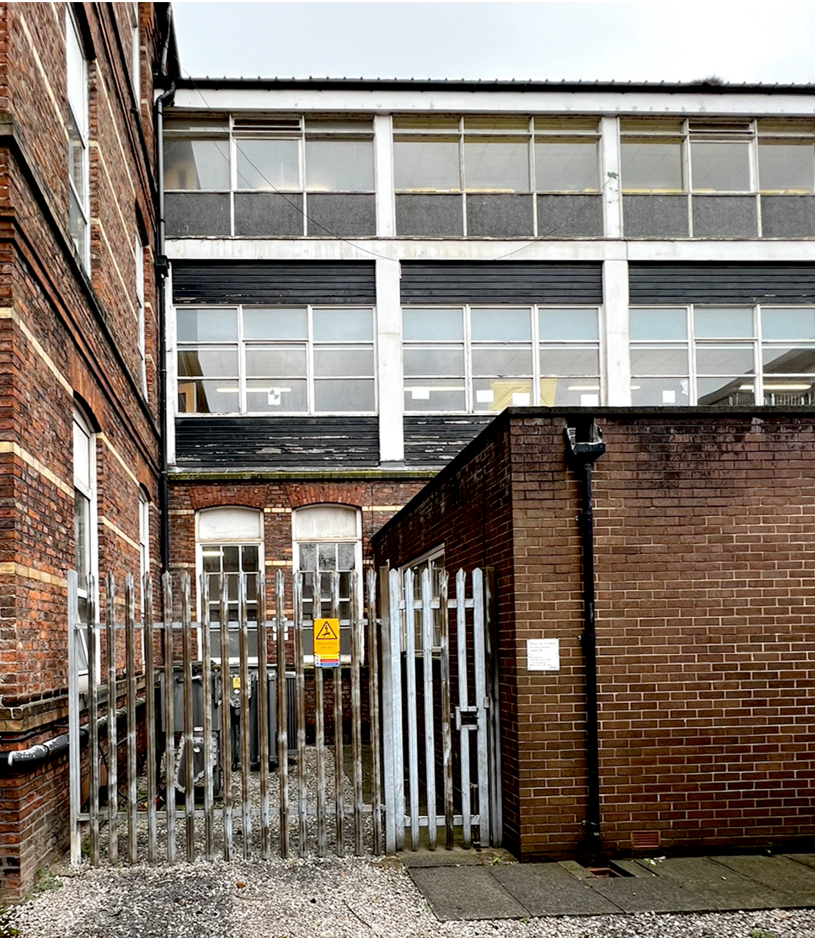
Figure 5: Image displaying existing Corridor Link cladding between Block B & Block C
