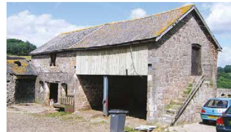
External steps mark the entrance to a granary sited above a 2-bay cartshed in the Oswestry Hills, attached to a stable. The whole range testifies to the intensification of arable farming in the mid 19th century in this upland area. Photo © Jeremy Lake
