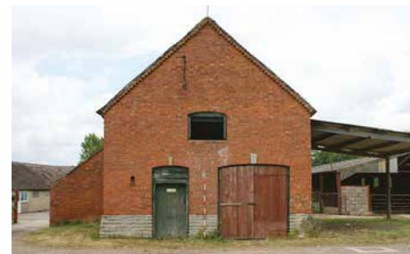
Coach houses can incorporate a stable, as here, and a first-floor loft for hay and/or for housing a stablehand. Photo © Worcestershire County Councils
