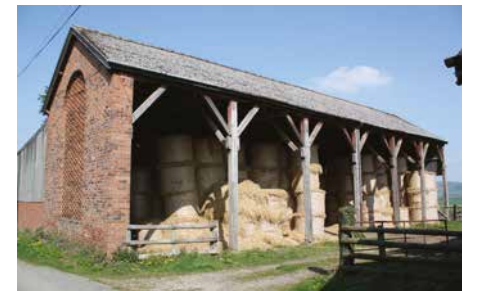
A mid-late 19th century hay barn on a planned farmstead built to house a large herd of dairy cattle, and the hay needed to feed them, in north Shropshire. Hay barns of this type, with brick piers or (as here) timber posts, are commonly associated with the large dairying farmsteads of this period found across the plains of Lancashire, Cheshire, Shropshire and Staffordshire. Photo © Jeremy Lake
