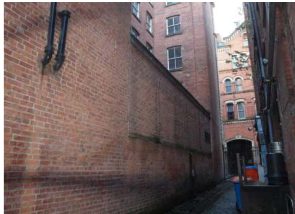
Image of the brickwork annex now demolished
