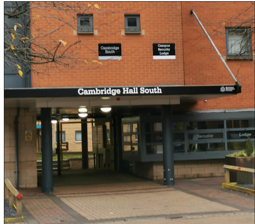
New sign installed
