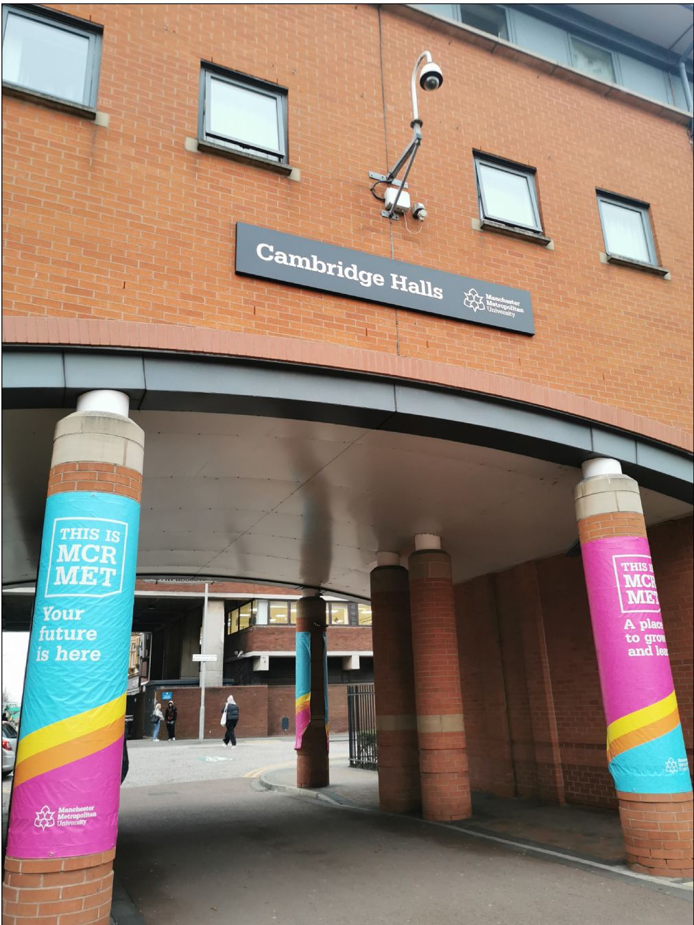
New sign installed
