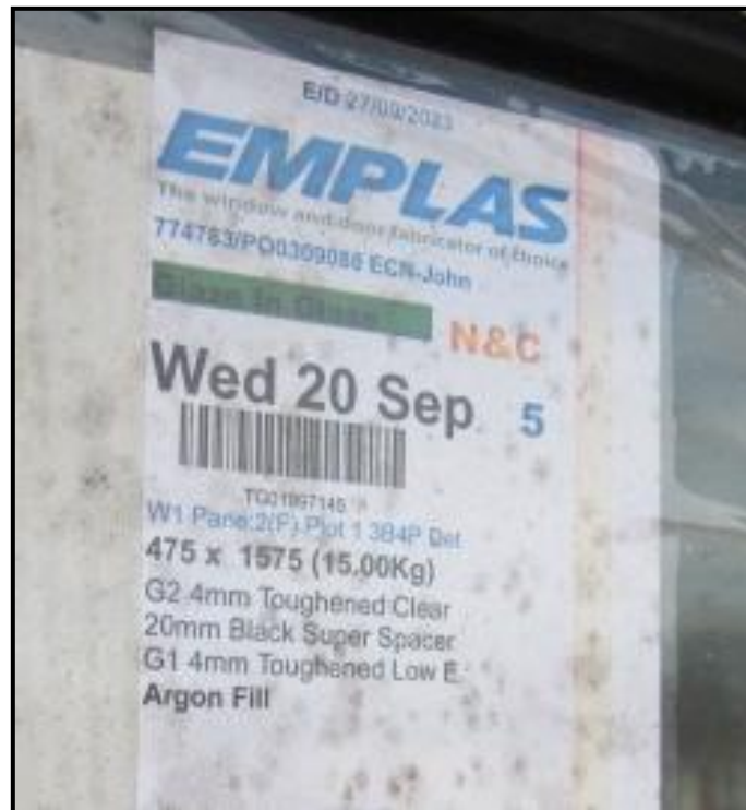
Photograph 6. Glazing sticker, front and rear bedrooms, plot 1
