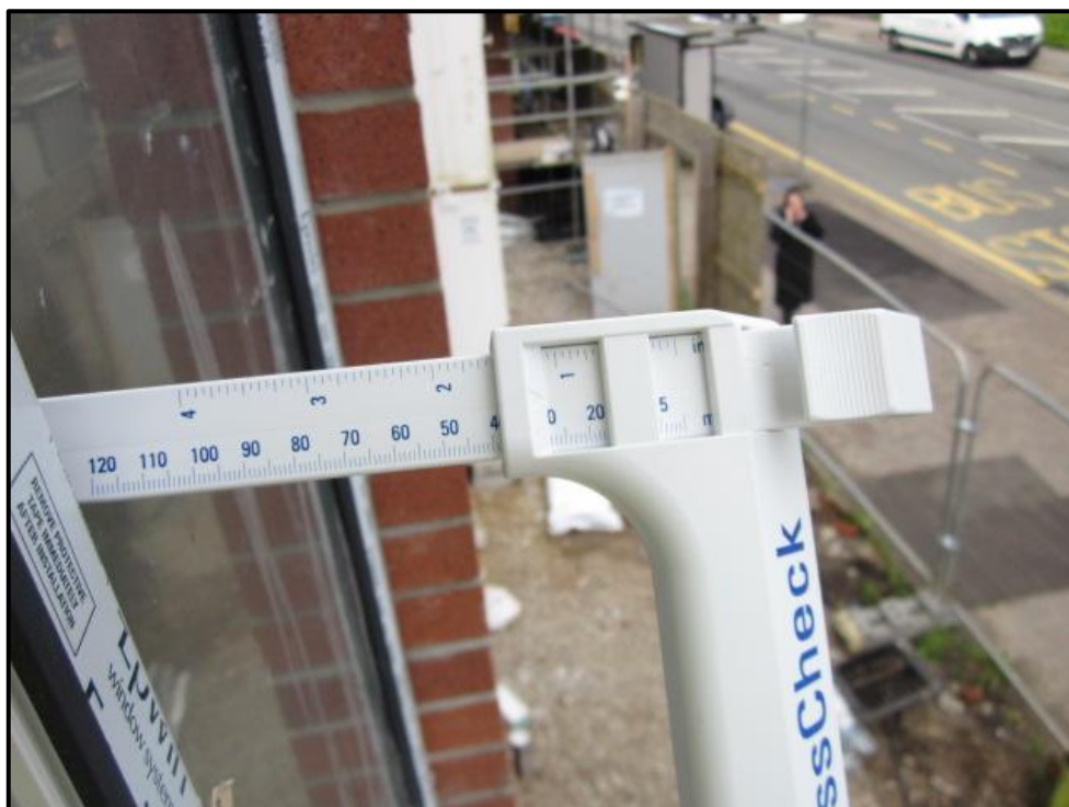
Photograph 7. Measured thickness of the sealed unit glazing, plot 1 - front bedroom
