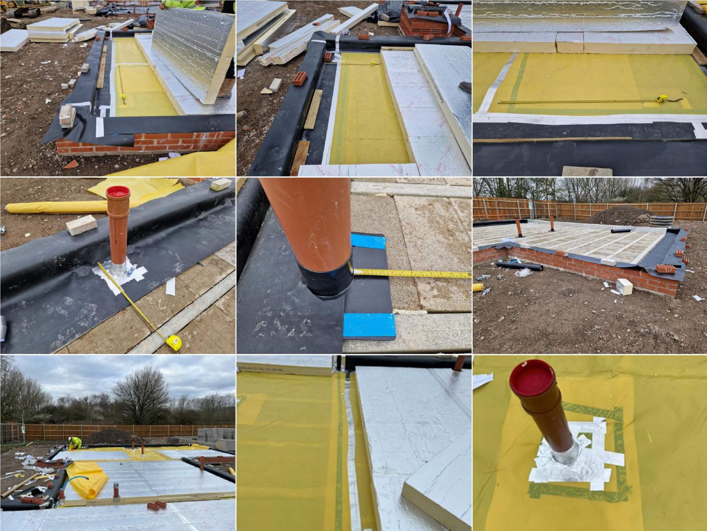
Visqueen Zedex Plot 9 showing Visqueen CO 2 membrane attached to Visqueen Zedex and preformed corners. EPS protection over the installation Visqueen Plot 9 Visqueen Membrane installed and lapped plot 9 Top hat service entry sealed through Zedex on Plot 10 awaiting membrane install. Beam and block floor can be seen Another top hat install on Plot 10 Zedex on plot 10 awaiting Membrane install Visqueen Membrane install on Plot 10 protected with EPS Visqueen Membrane installed and lapped plot 10 Complete sealed service entry on plot 10 with laps
