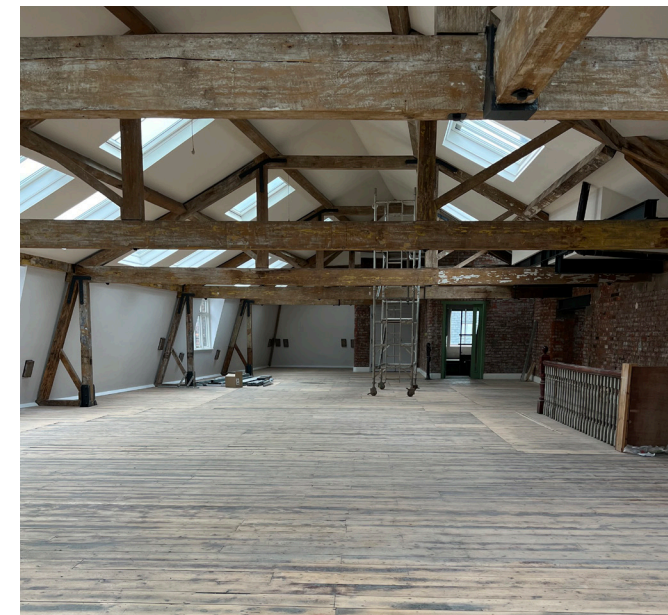
Image 10: Photograph of fourth floor, with stairs and exposed timber flooring.
