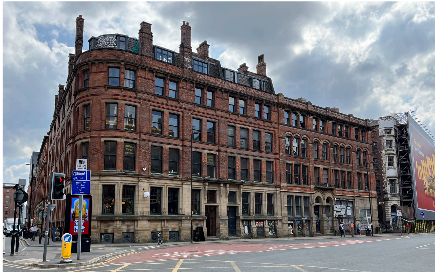
Image 1: Photograph of site, taken from corner of Newton Street and Dale Street, April 2024.
