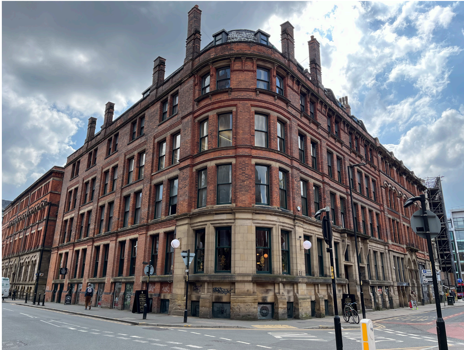
Image: Photograph of site, taken from corner of Newton Street and Dale Street, April 2024.
