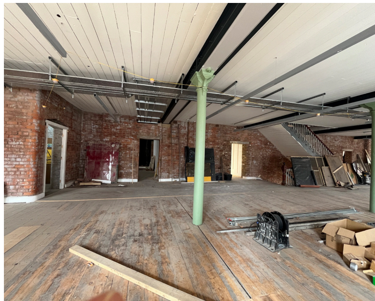
Image 8: Photograph of third floor, showing original brick walls and stairs in area of proposal.
