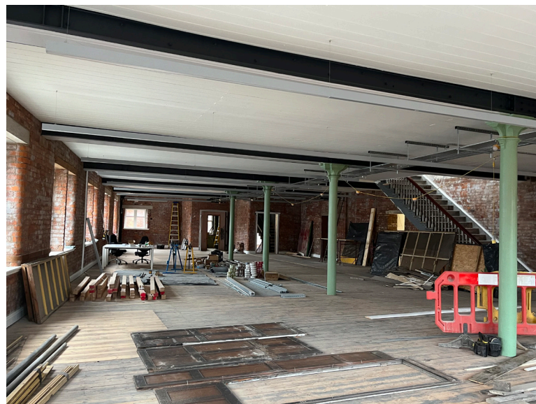
Image 9: Photograph of third floor showing columns and timber flooring.
