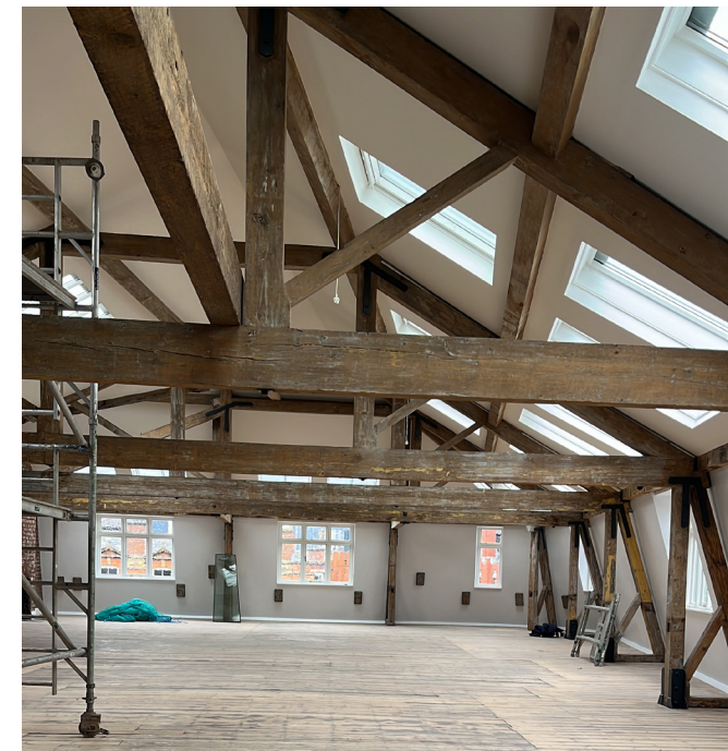
Image 11: Photograph of fourth floor, showing exposed roof structure.
